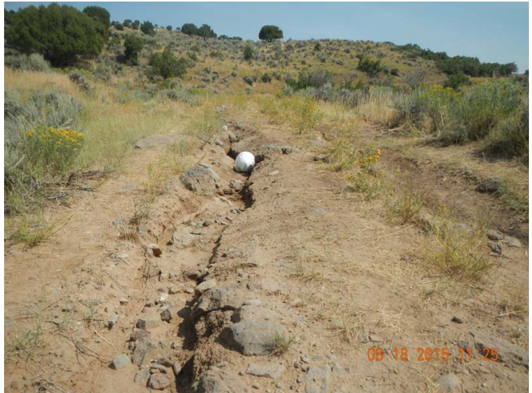
Rill in access road. Evidence of sediment and coarse material being transported. Hard hat for scale.
