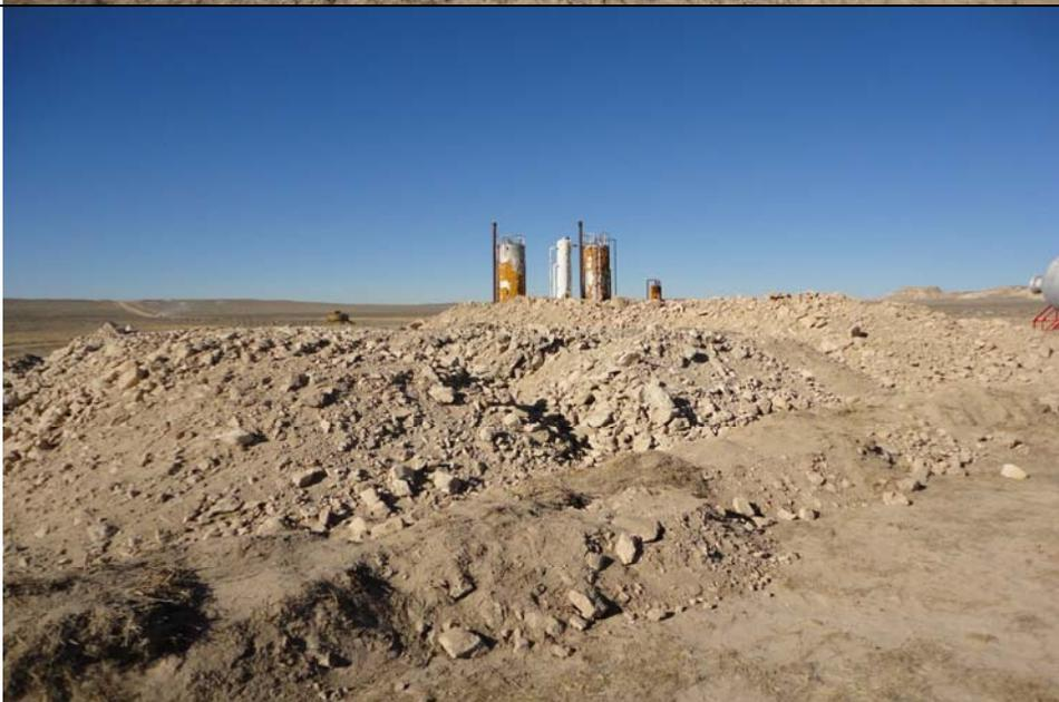
**Subject:** Southwest corner of the land farm stock pile. The materials on the north and south side of the stock piles contained more rock and did not have as much staining as those in the center of the pile. These materials may be able to be sampled and used to finish backfilling the first pit (COGCC ID#100036) located beyond the vertical separators in the background and on the west end of the Terrace Gas Plant.
