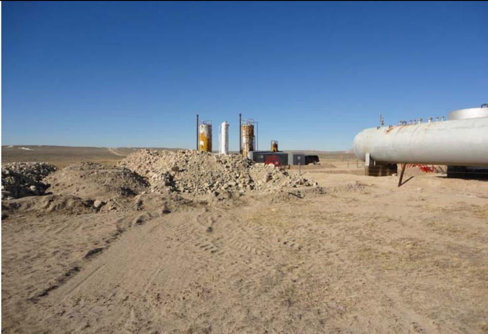
**Subject:** Materials on the north side of the stock pile were also more rocky and were excavated from the first pit on the west end of the Terrace Gas Plant. The materials are rocky with some large bedrock pieces, and did not appear to be heavily stained. It may be possible to remove some of this material for use in backfilling the first pit pending sampling and analysis.
