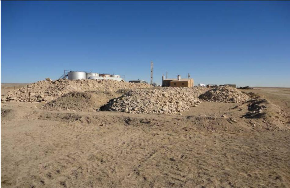
**Subject:** Land farm stockpiles – west side of containment berm located south of the Terrace Gas Plant and WCR 118. The berm measured 68 feet North – South and was approximately 1.5 feet in height.
