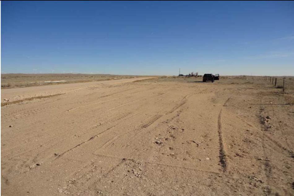
**Subject:** Photograph shows the location of the second pit, COGCC ID# 100035, located approximately 800 feet to the west of the Terrace Gas Plant. K&K reclaimed the pit using fill material from the Nelson Ranches gravel pit to the west. The area needs to be re-seeded to finish the reclamation.
