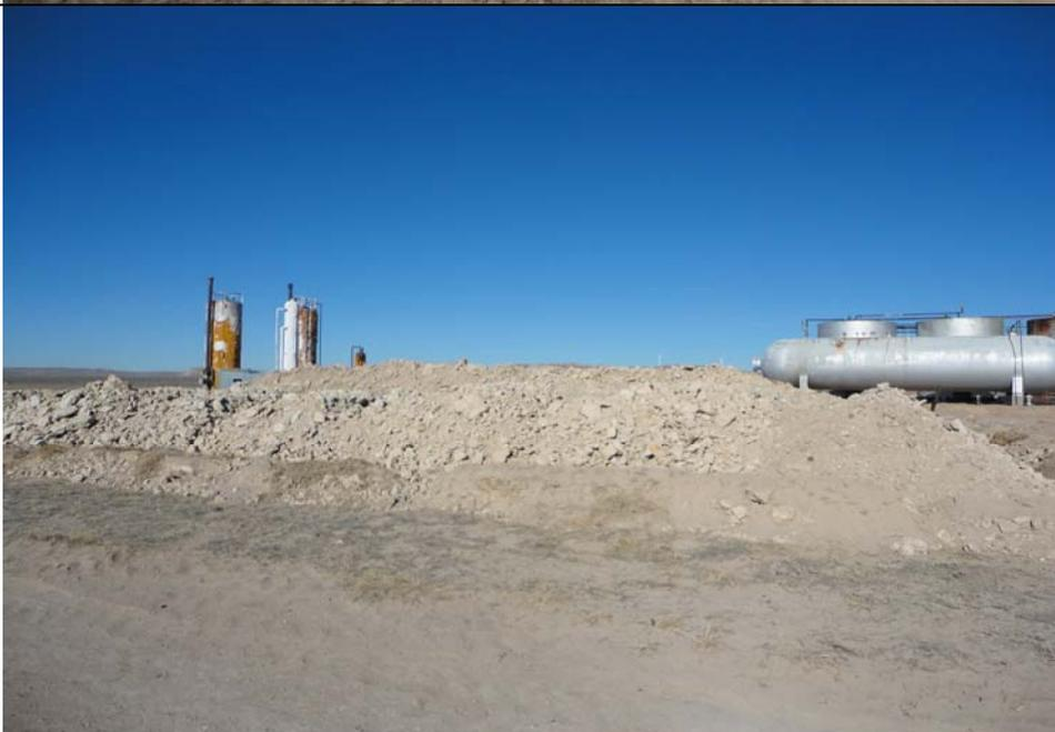
**Subject:** South side of the land farm stockpile containment. Material on the south side of the containment was more rocky and not as stained as material in the center of the containment.
