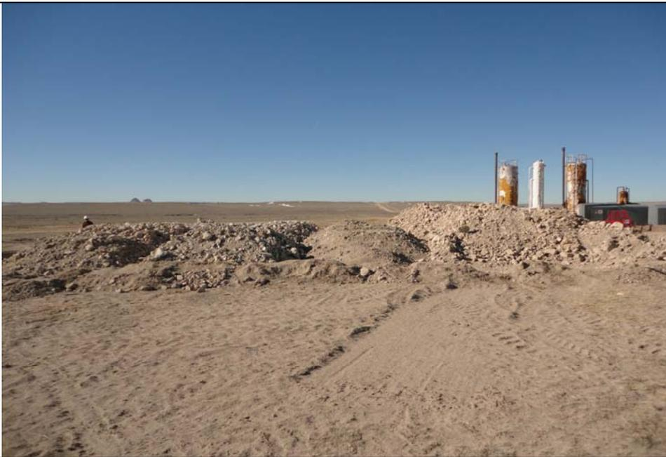
**Subject:** East side of land farm soil stock pile and earthen containment berm. Stained material in the center of the berm area was stock piled in piles that were approximately 4 feet in height. Materials on the north side of the stock pile were approximately 8 feet in height.
