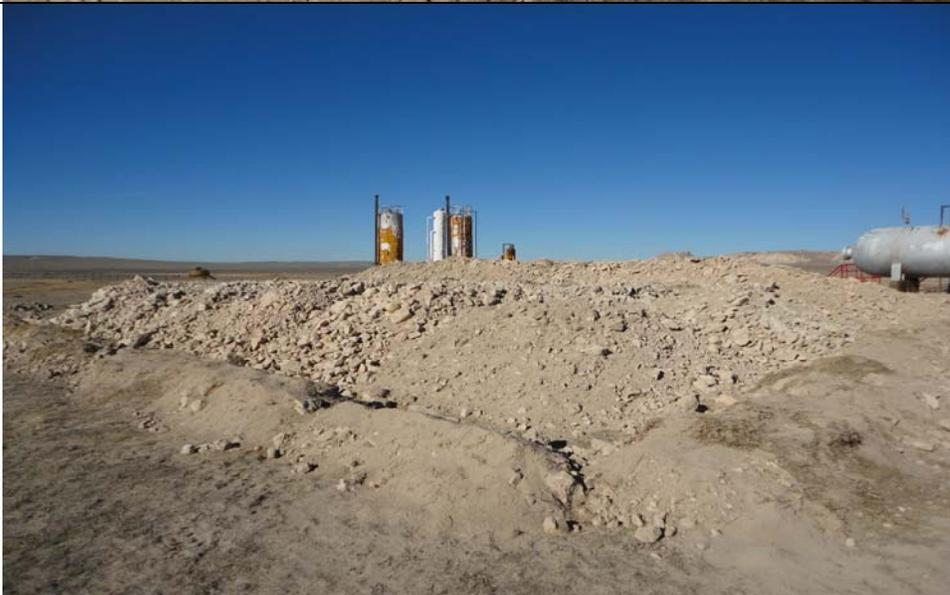
**Subject:** Southeast corner of the land farm stockpile. The earthen berm measured 100 feet east-west and was approximately 1.5 feet in height. The earthen containment berm had some areas which need to be built up.
