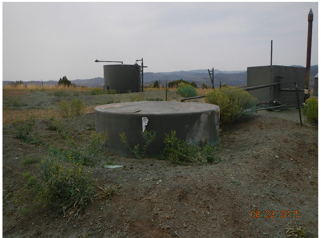
Vegetation in tank containment. Peeled label.
