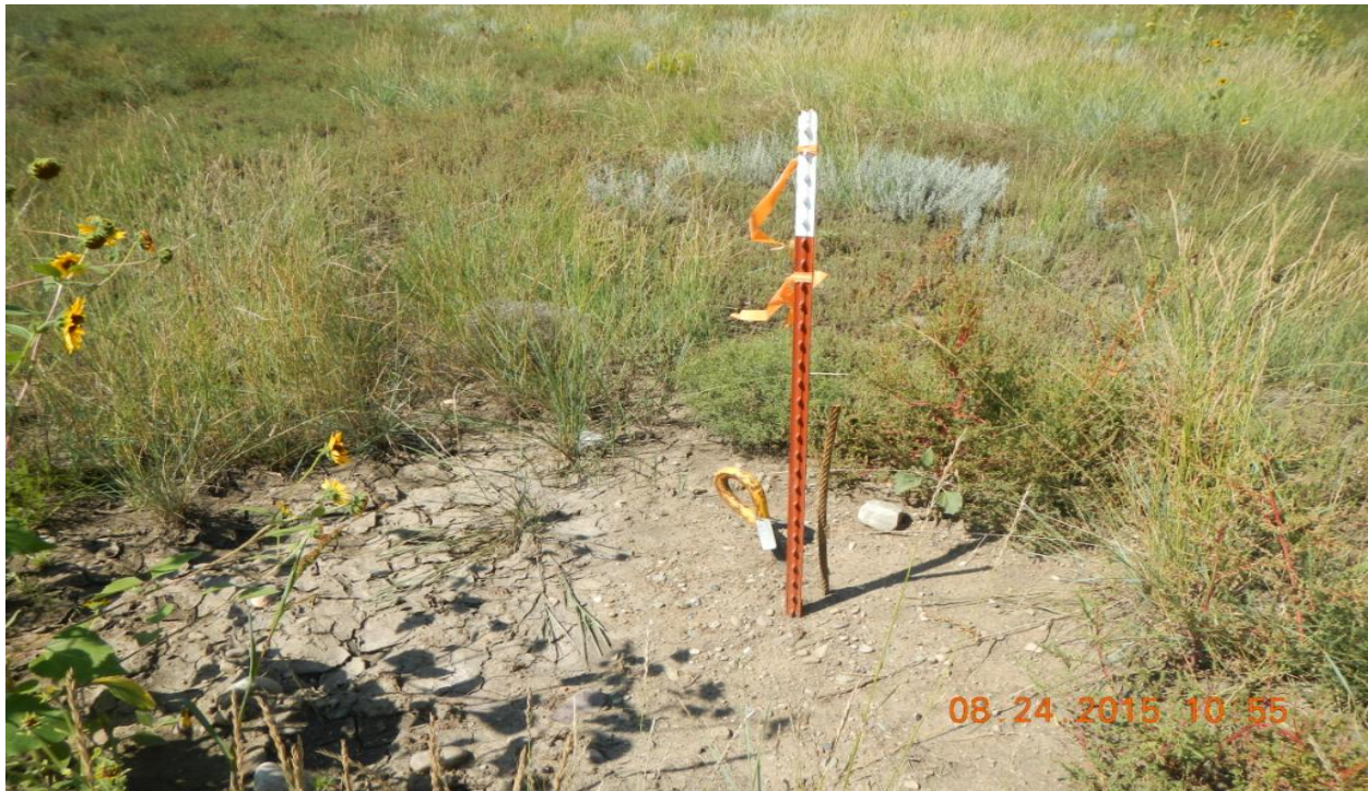
photo 5: Guy line anchors are properly marked.
