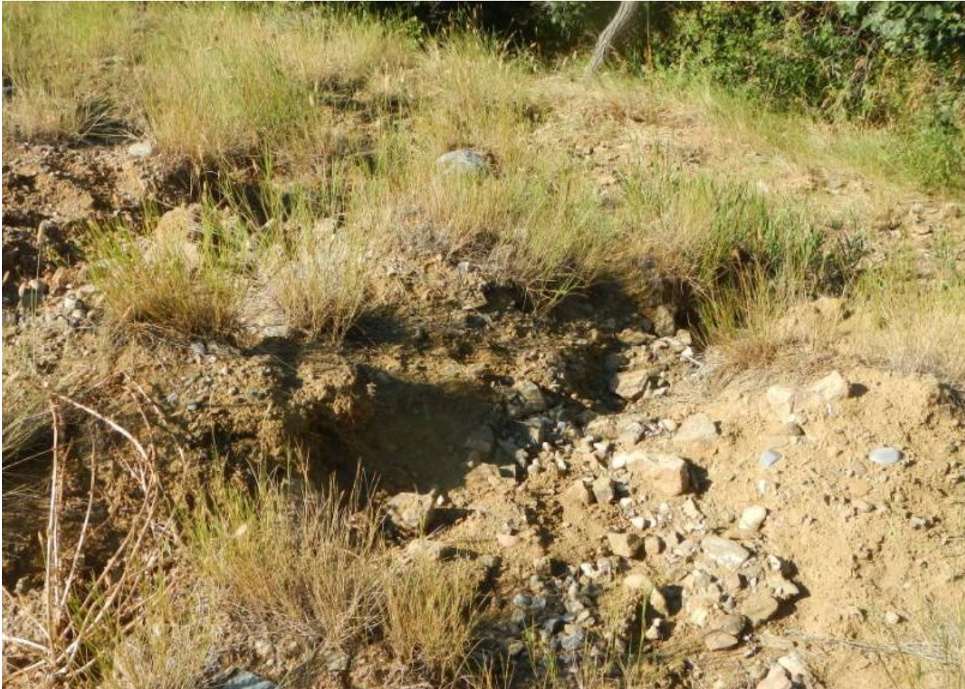
Photo 1. View of erosional channel (approximately 15 inches wide and 10 to 12 inches deep) forming within the western portion of the project area from the southwestern edge of the working area facing down-slope.
