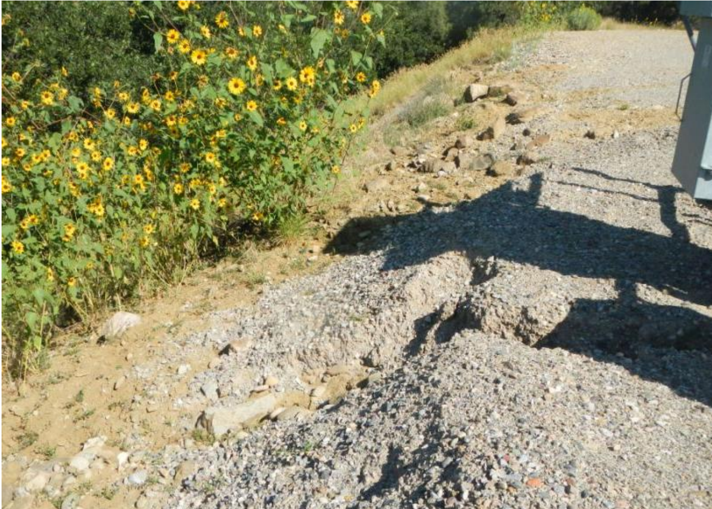
Photo 3. View of erosion along western edge of well pad where stormwater flows are eroding the western edge of the well pad.
