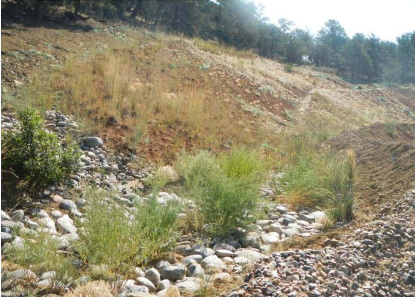
Photo 4. View of revegetation progressing on the tall, cut slope in eastern portion of the project area. Stormwater BMP in foreground appears to be functioning to de-energize stormwater flows coming off of the eastern cut-slope.
