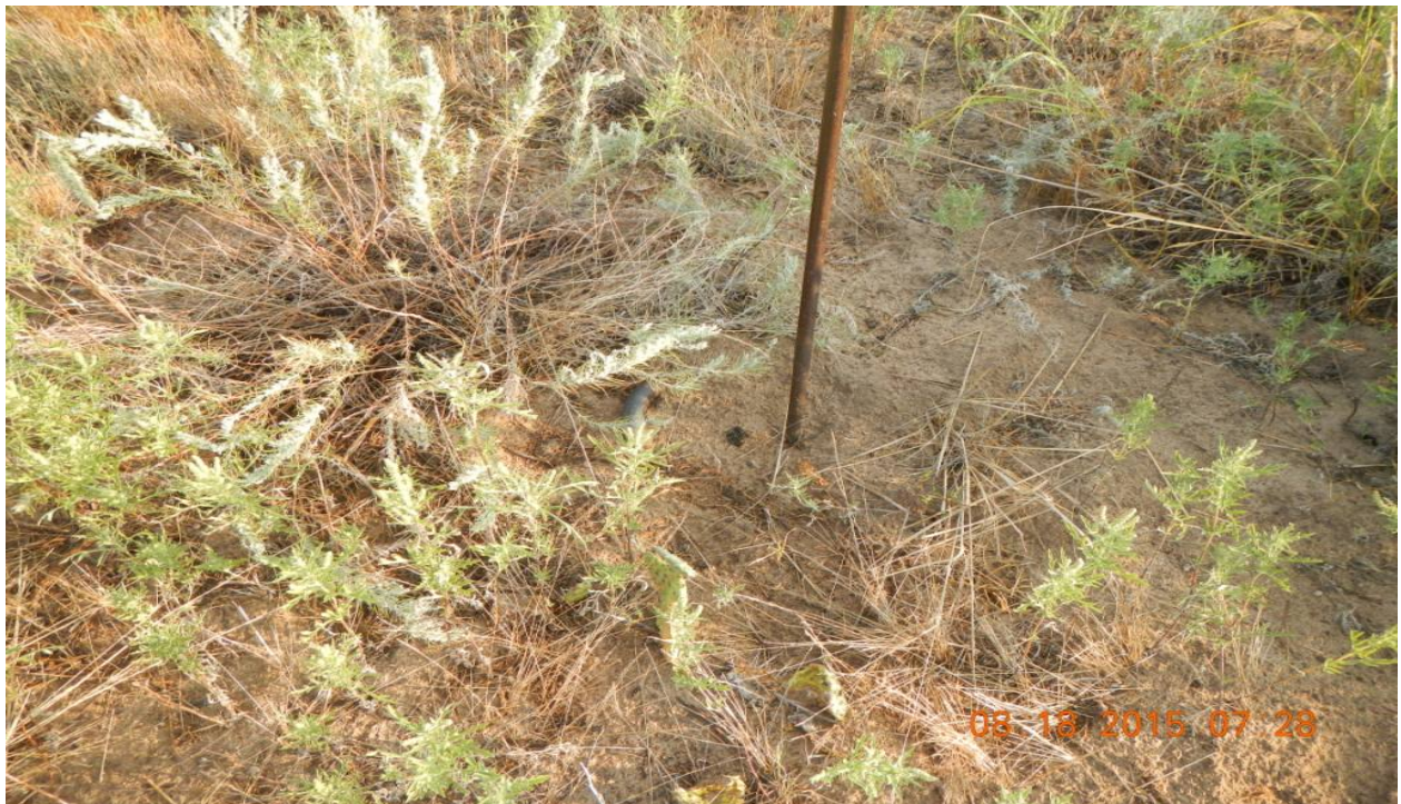
photo 6: Close up of the guy line anchor which has not been removed.
