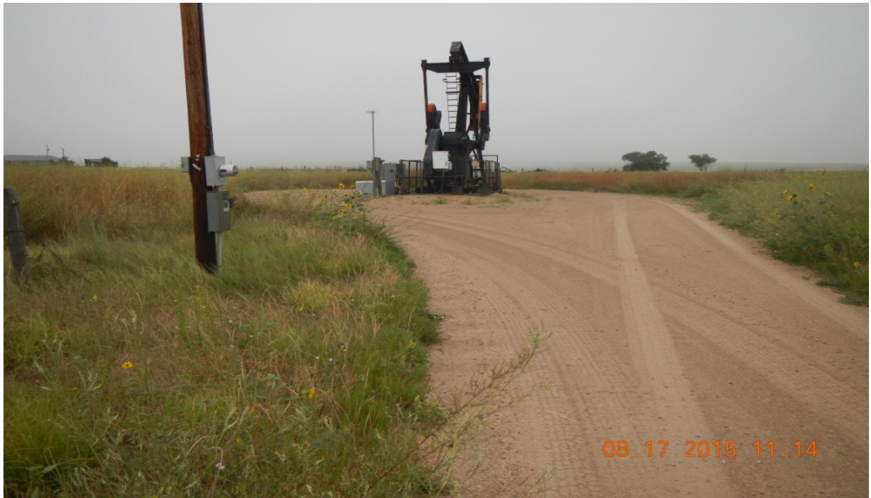
photo 3: Facing west towards the equipment at the location.
