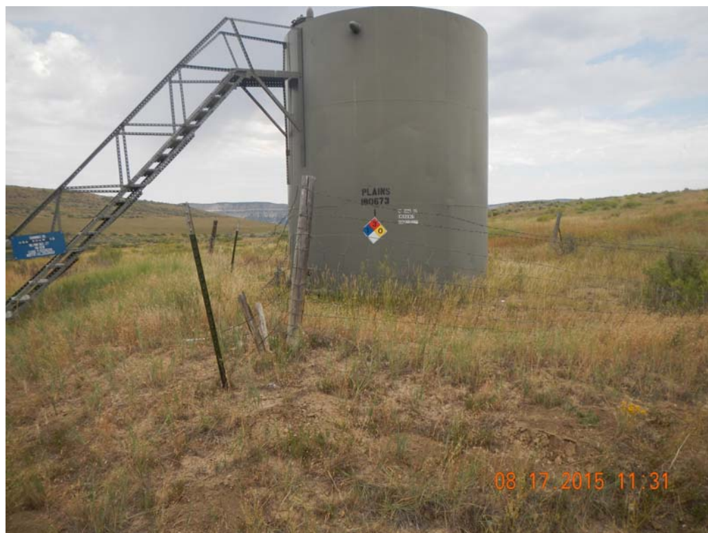
Incomplete tank label. Overgrown berm. Fence falling down.
