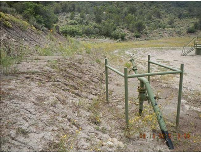
RUN ON CONTROL BERM ON EAST SIDE WELL PAD FULL OF SEDIMENT; CUT SLOPE EROSION FORMING UNDER UNMAINTAINED BMP.
