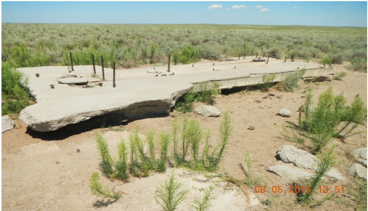
photo 3: Concrete slab approximately 18'x10'x2' in size.
