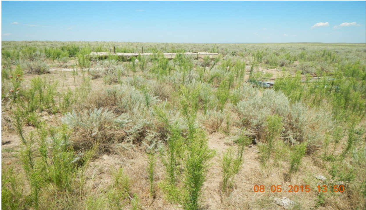
photo 1: Facing northeast towards location where debris, trash, and concrete slab remains.
