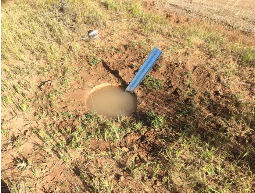
Figure 1. Valve can that overflowed due to a gas eliminator failure causing 1bbl of produced water to spill onto the pipeline ROW. A vac truck pulled standing water from the valve can. Spill area is 7' x 7'.
