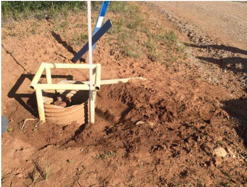
Figure 2. Valve can that overflowed due to a gas eliminator failure causing 2 bbls to spill onto the pipeline ROW and borrow ditch. Spill area is 15' x 5'.
