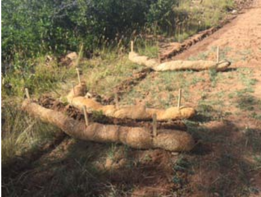
Figure 7. Straw wattles placed at the terminus of the spill path. Looking up the spill path.
