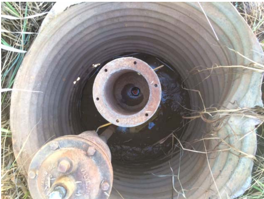
Figure 2. Valve can with the gas eliminator that failed causing 6 bbls to leak into the borrow ditch.
