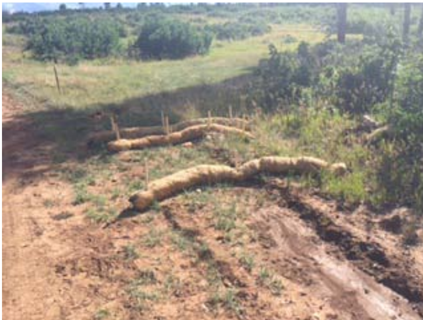
Figure 8. Straw wattles placed at the terminus of the spill path. Looking down the spill path.
