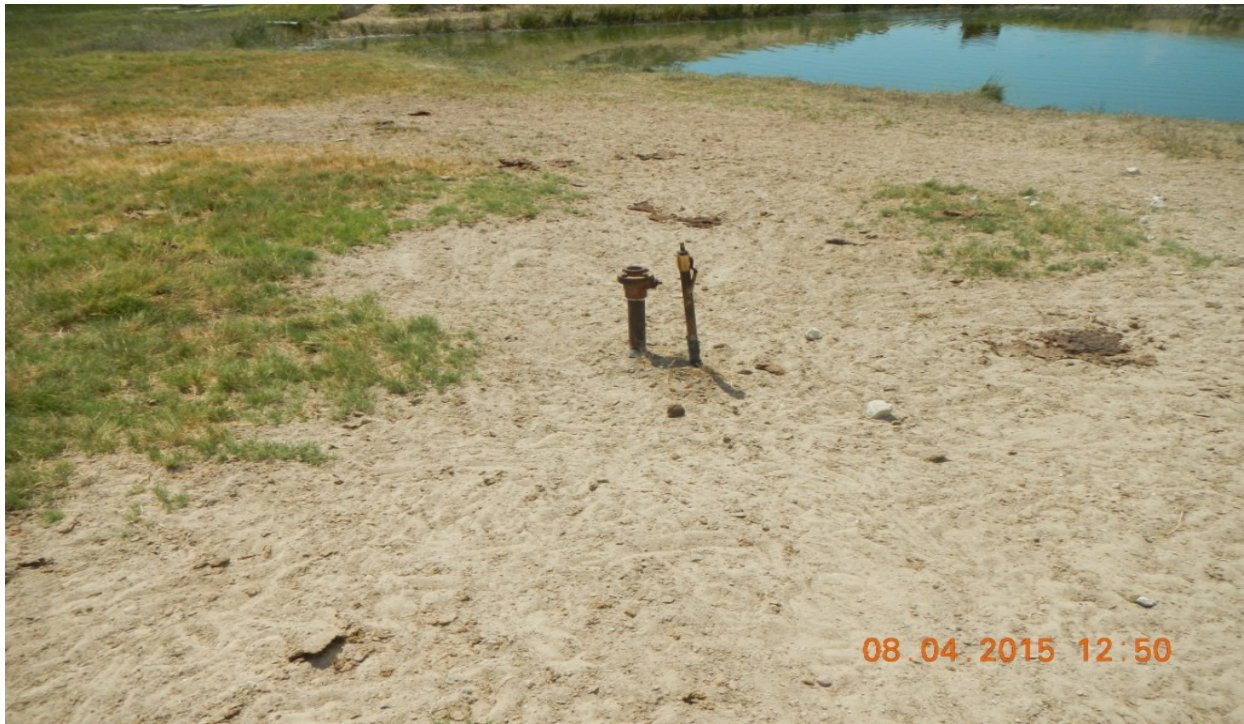
photo 9: Pipe riser found at center of the location. Lat:40.288/Long:-104.637
