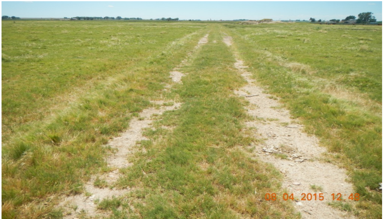
photo 2: Facing south towards the location. Access road has not been recontored and reclaimed.
