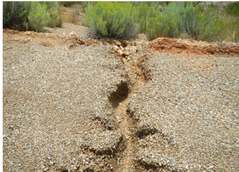
Photo 4. View of erosional feature forming within eastern portion of well pad.
