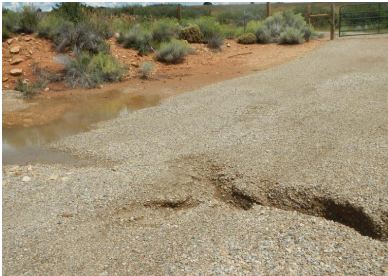
Photo 4. View of erosional feature forming within eastern portion of well pad.
