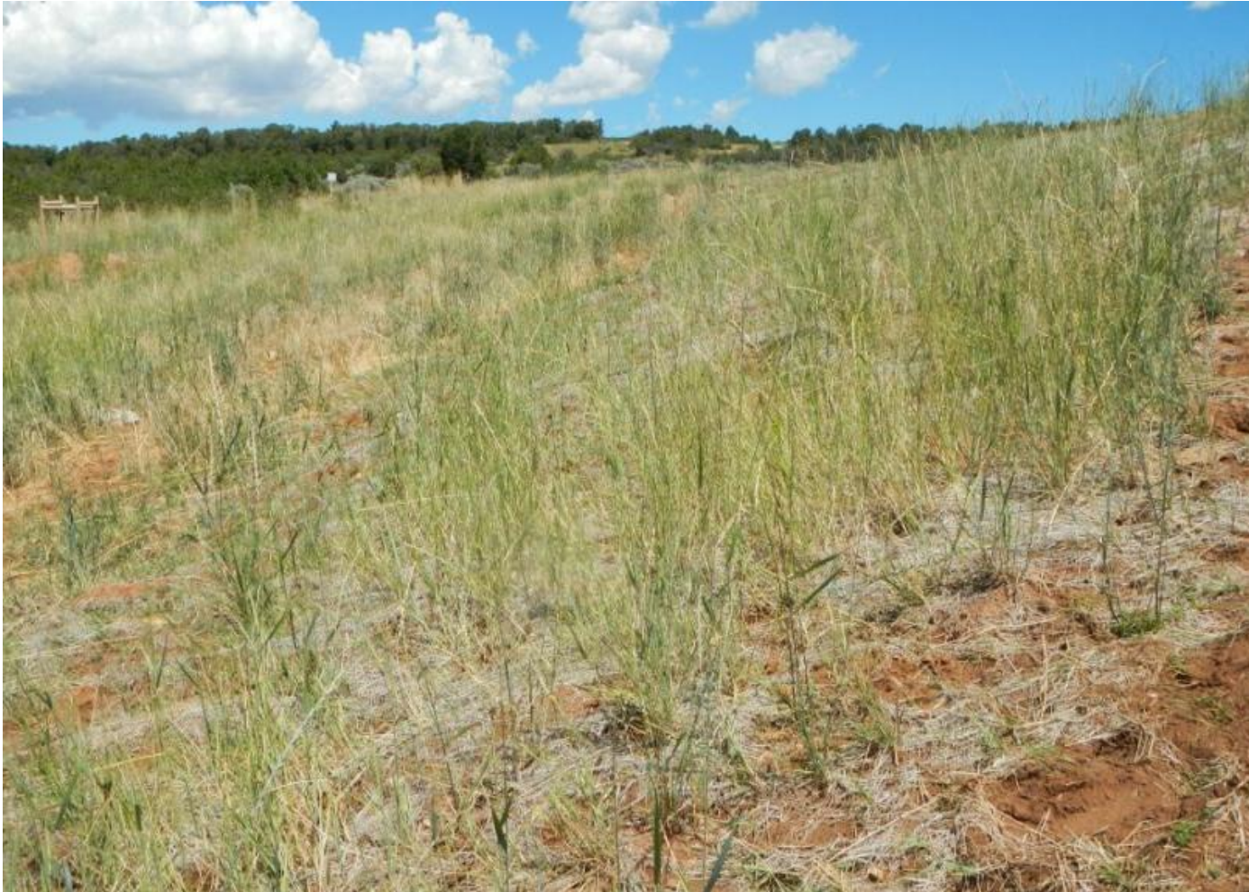
Photo 4. View of western portion of project area from southwestern corner facing northward. Good revegetation along this slope.
