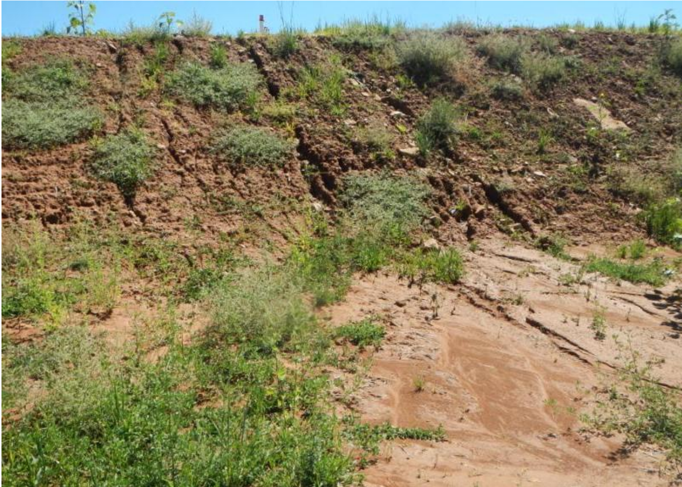
Photo 4. View of rill erosion and sediment deposition in western portion of project area.
