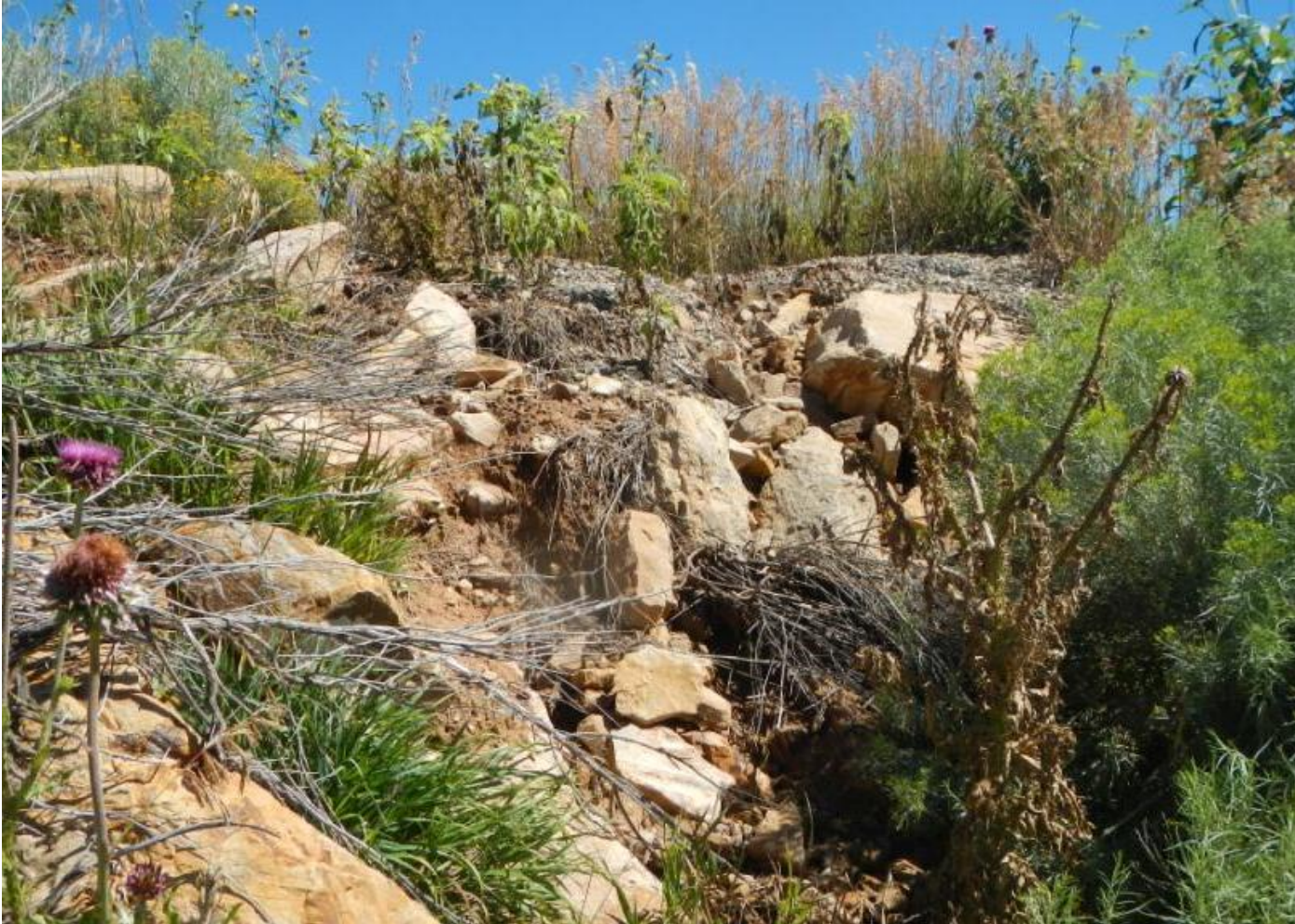
Photo 3. View of area where stormwater flows have eroded a portion of the southern fill slopes on the well pad.
