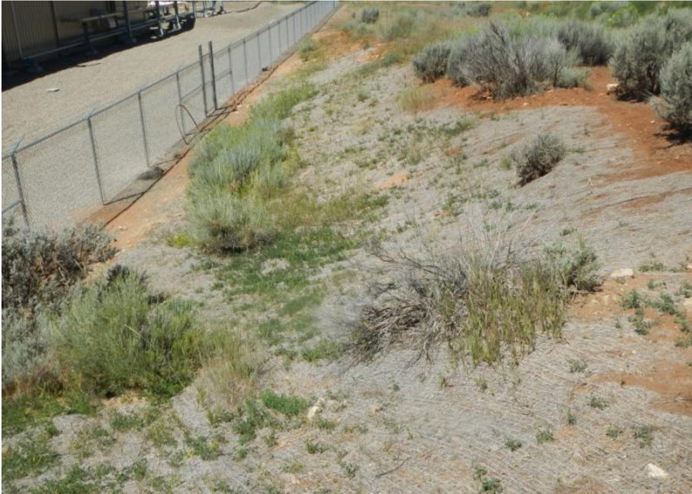
Photo 7. View of cut-slope along northeastern portion of the project area. Straw matting and vegetation appear to be effective at stabilizing this slope.
