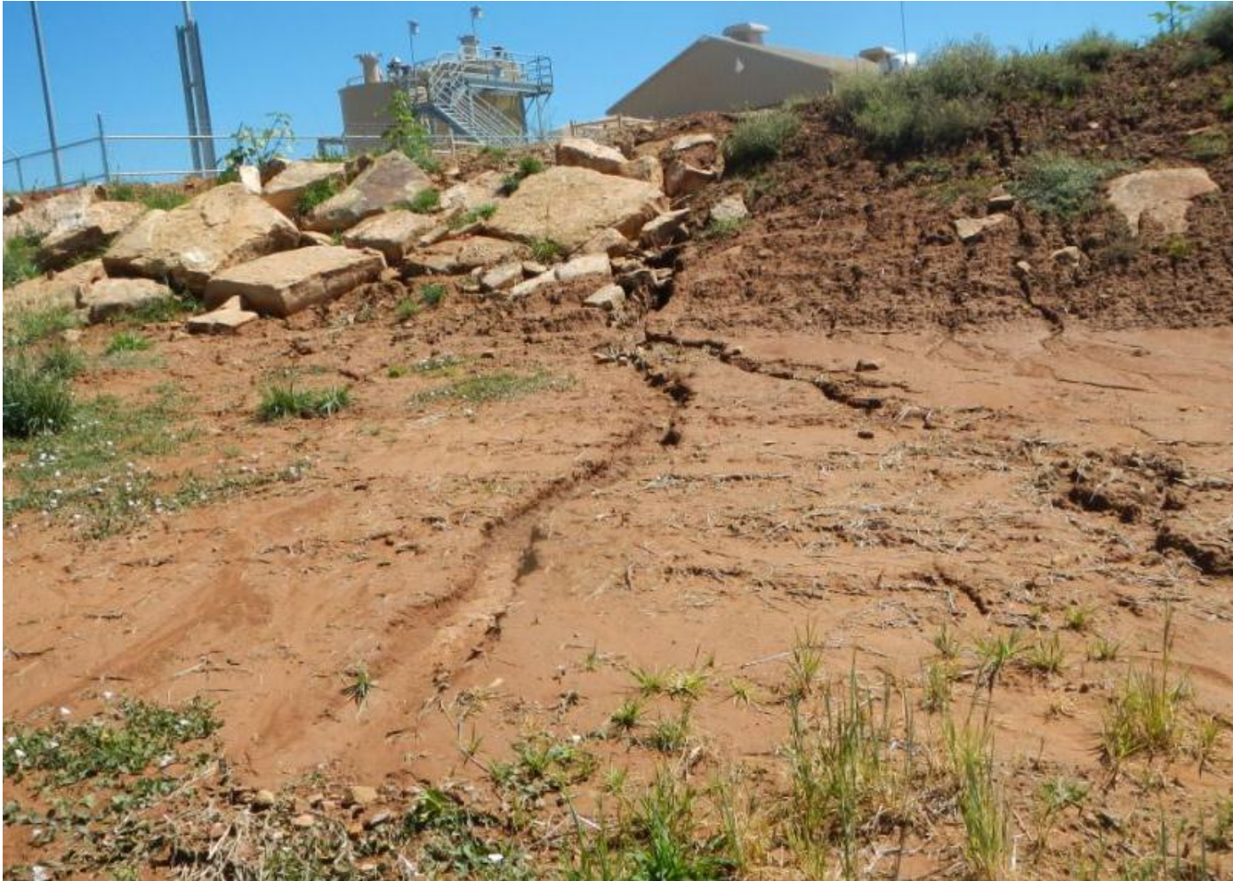
Photo 5. View of deep rills and sediment deposition within the western portion of the project area.
