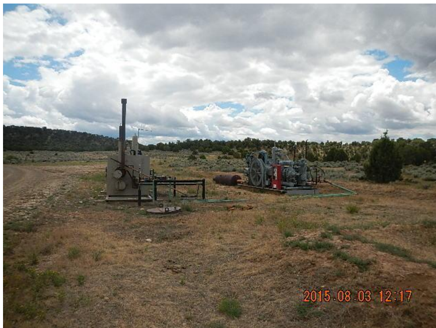
Horizontal heated separator, gas meter, and compressor on remote location
