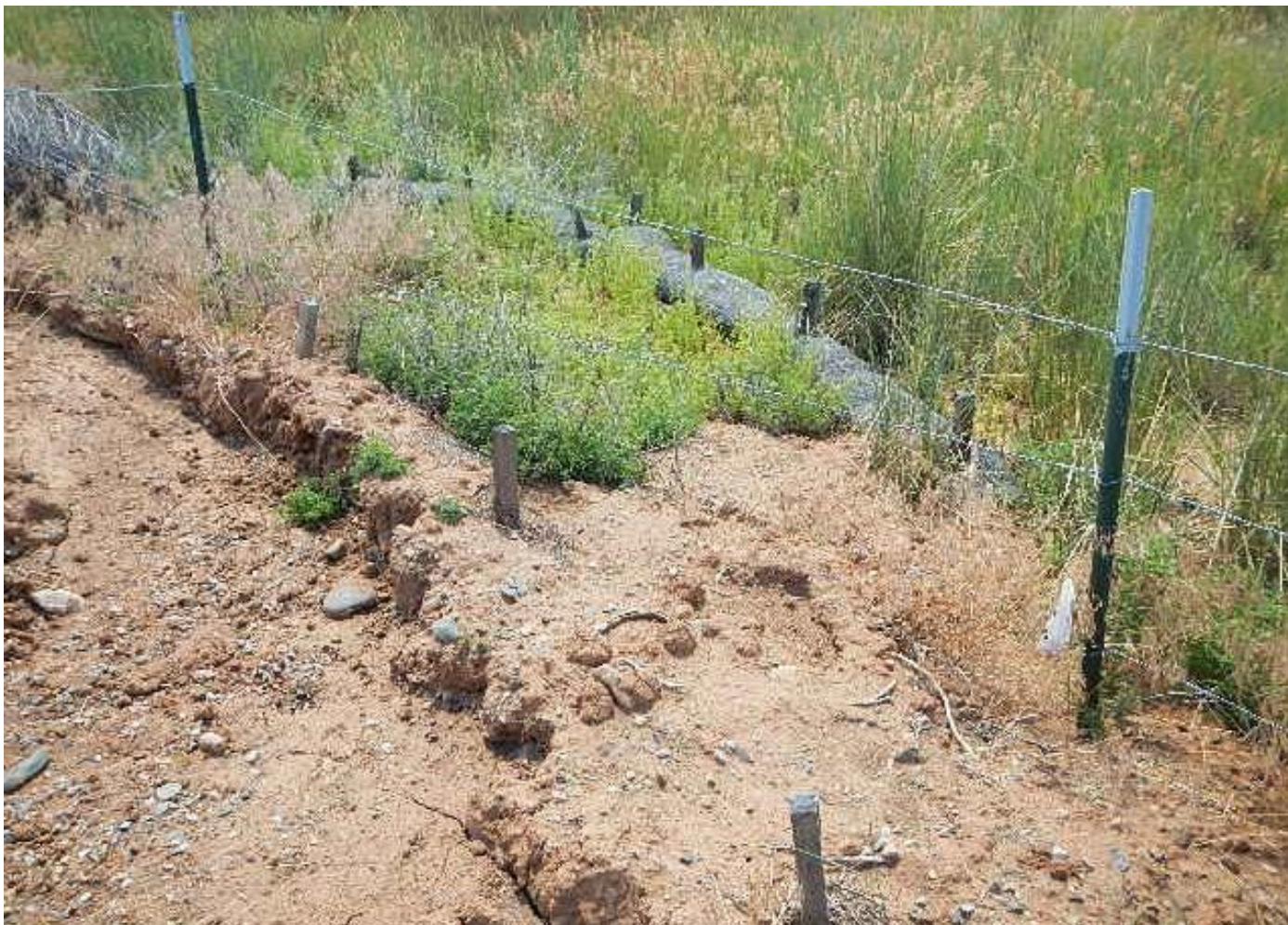
Photo 2. View of sediment overflowing straw wattle that is contained by second wattle. This needs maintenance and needs to be monitored.
