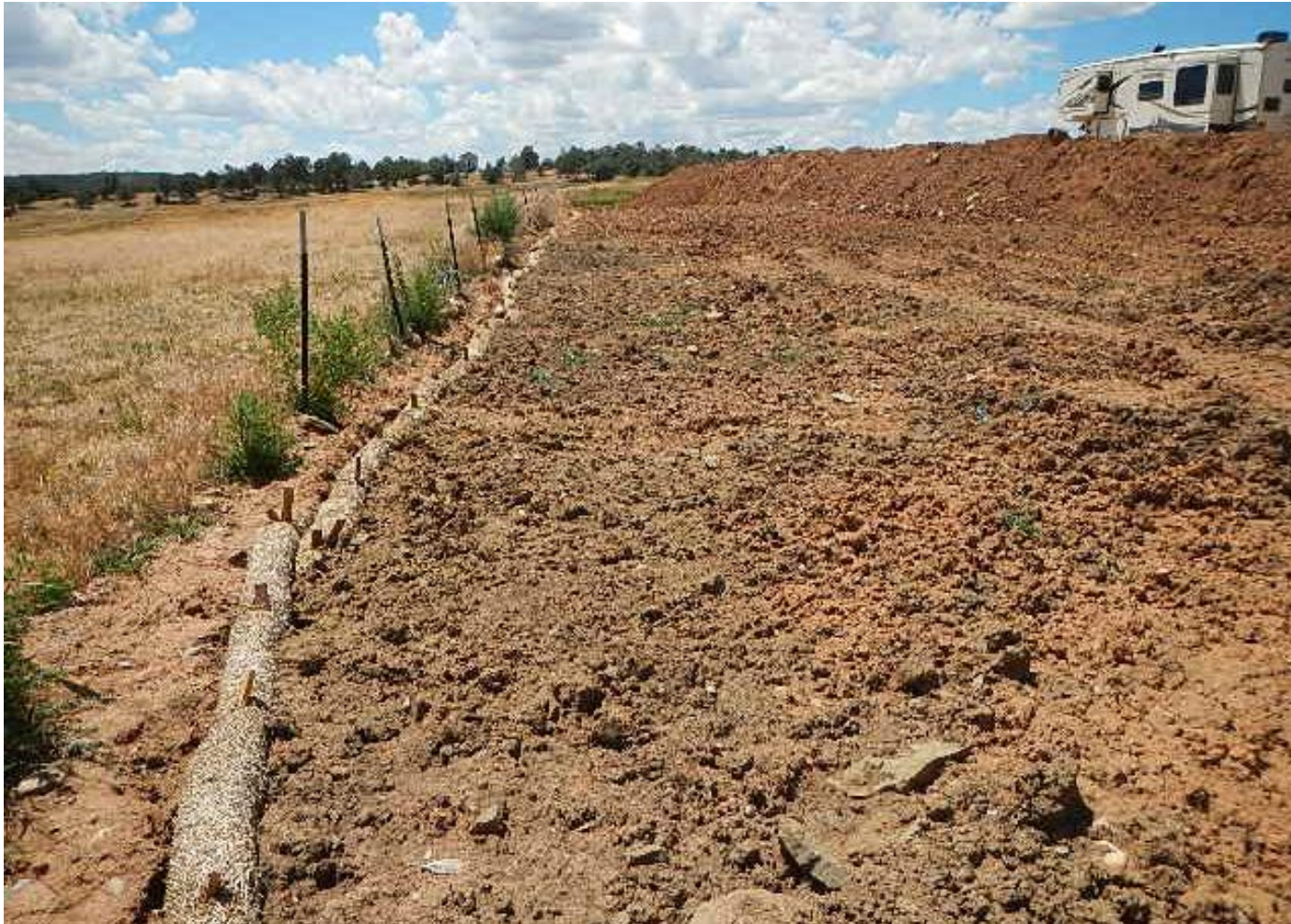
Photo 4. View of southern portion of project area from southeastern corner facing westward. Wattles appear to be properly installed and soil stockpiles are set back from edge of project area.
