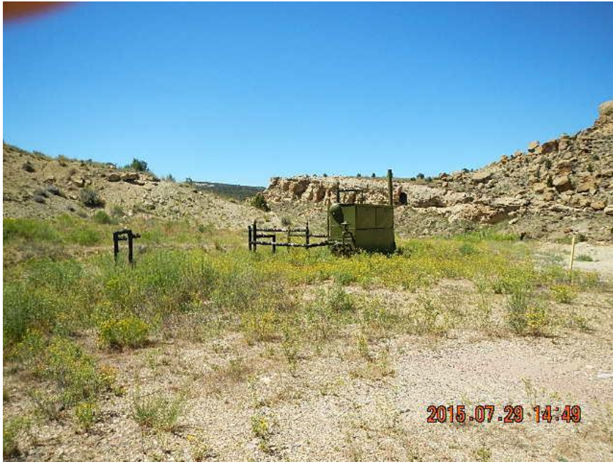
Brush/weeds within 25' of production equipment.
