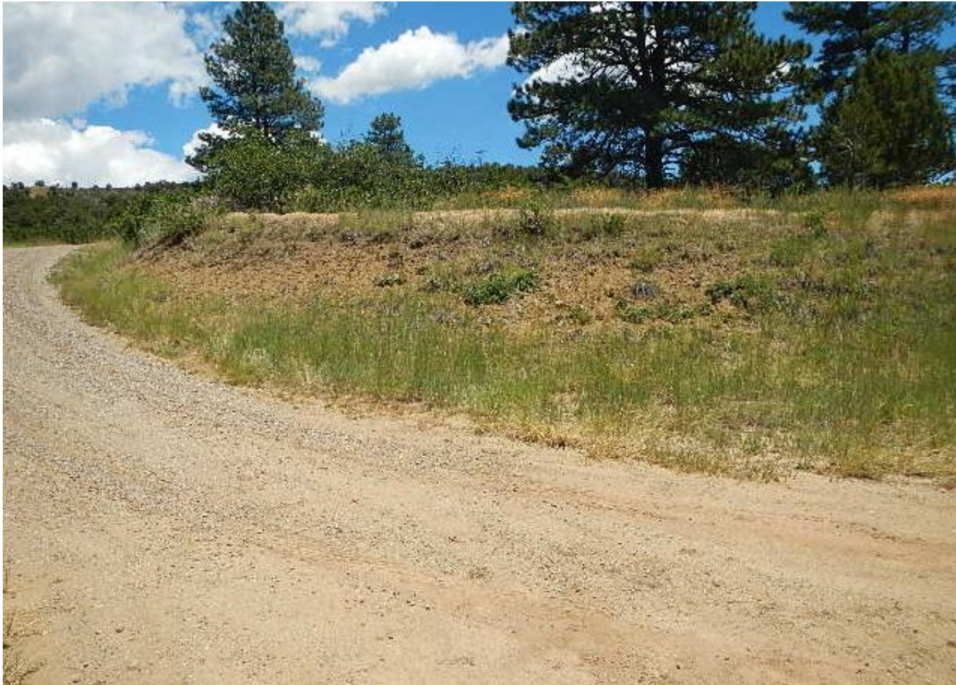
Photo 1. View of southern portion of access road facing southeastward.
