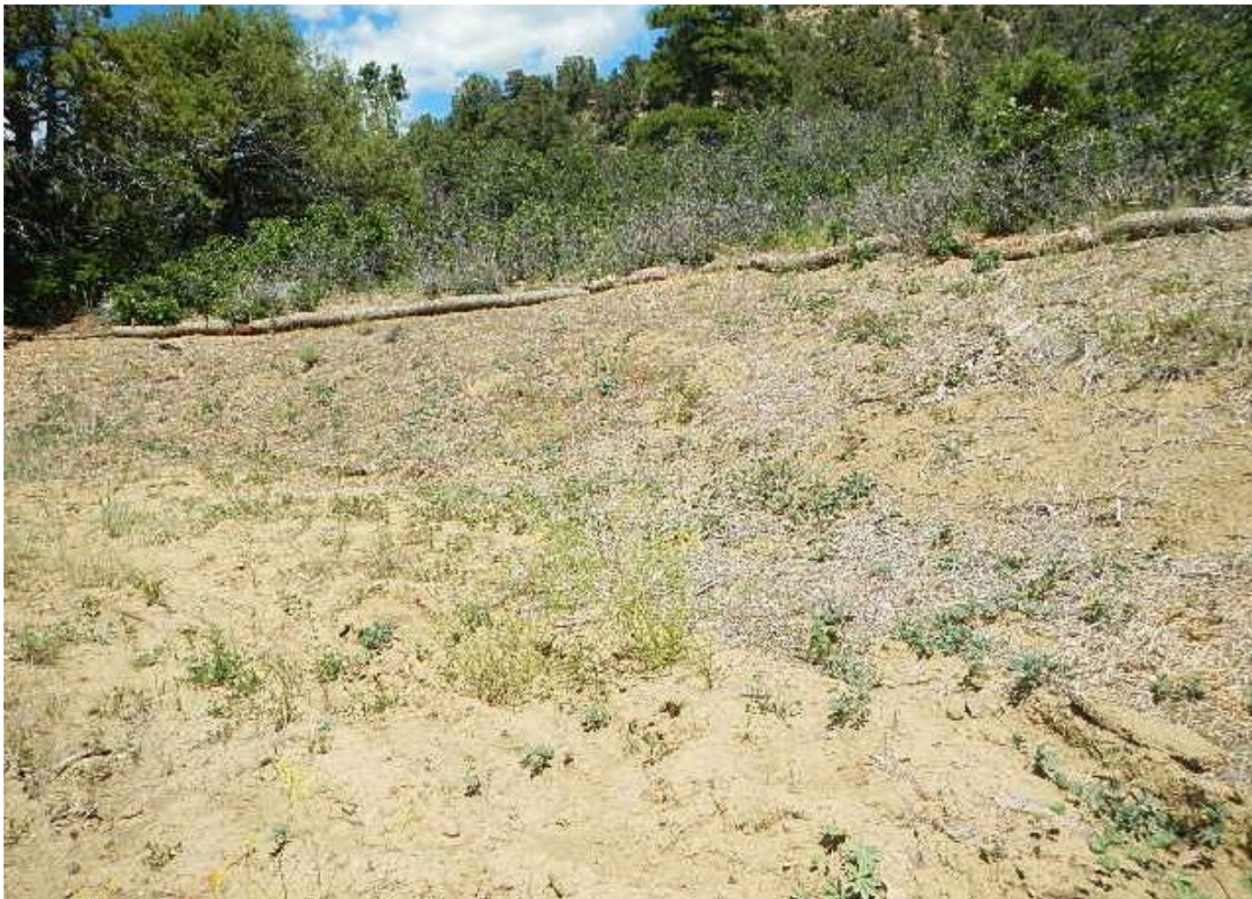
Photo 2. View of straw wattle and straw mulch in northeastern corner of project area. These appear to be stabilizing erosion at this time.
