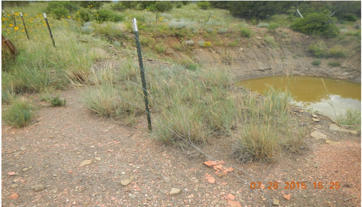
photo 5: Fence around the pit is down and not maintained.
