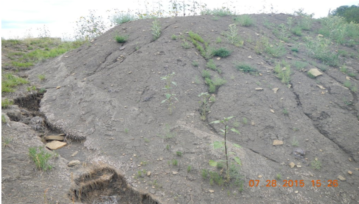
photo 10: Southeast side of the location has signs of erosion and minimal vegetation growth.
