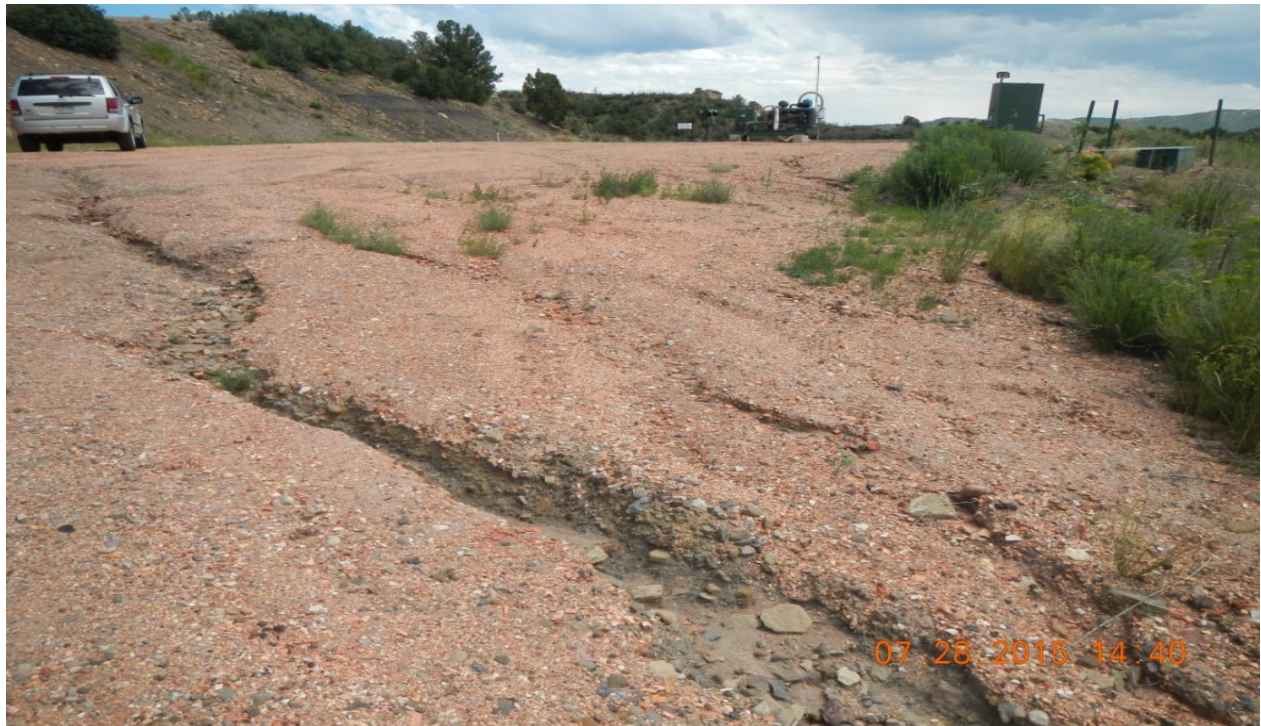
photo 3: Facing southeast towards the location. Erosion channels have developed transporting sediment off the location.
