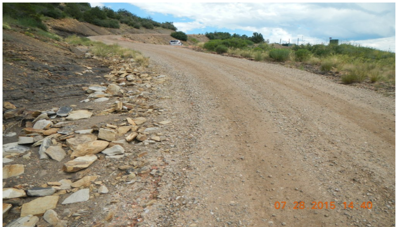
photo 2: Facing east along the main access road towards the location. Erosion is occurring along the side of the road.
