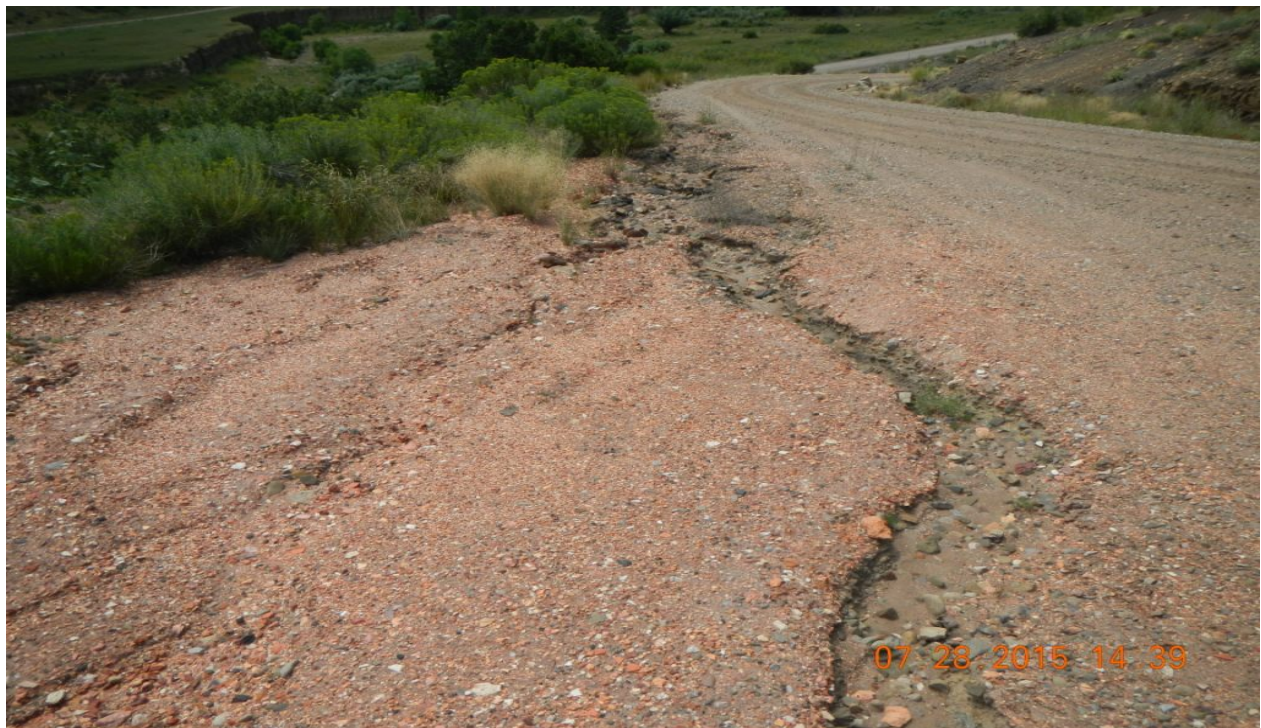
photo 4: Facing west at edge of location near the main access road. Erosion channels are shown.
