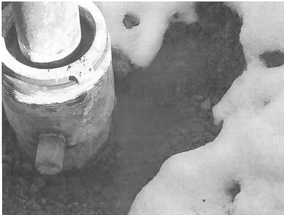
Photo 2: Methane seepage next to surface casing for Flagg #6-3 production well.
