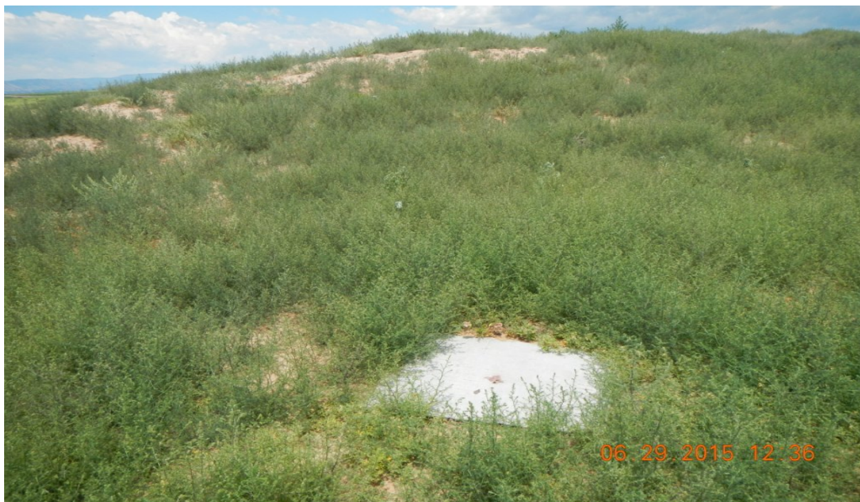
photo 9: Debris found at the south side of the dirt pile.
