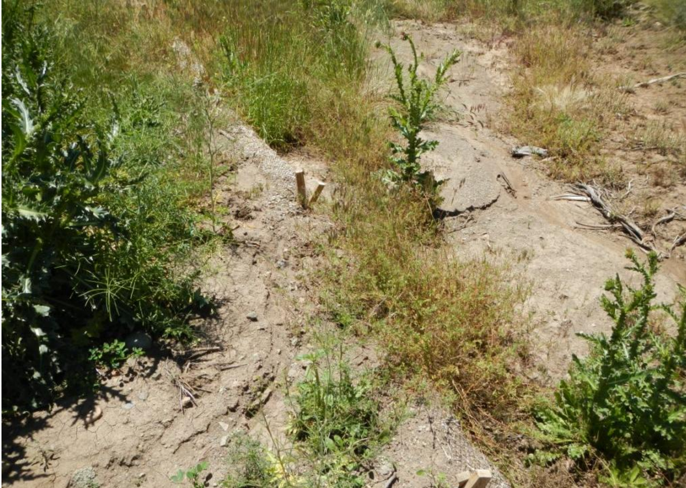
Photo 4. View of sediment deposition along western edge of project area showing where sediment appears to be discharging outside of the project area straw wattles.
