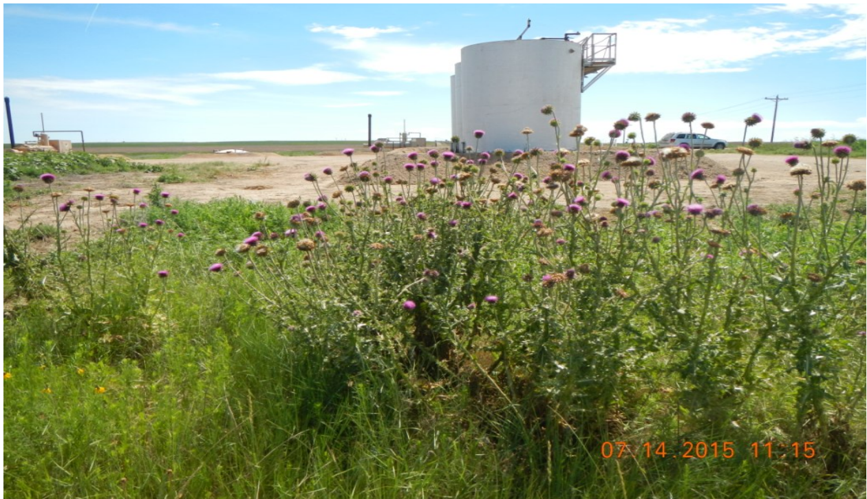
photo 4: Northwest side of the location. Weeds (Musk thistle) found growing around the location.
