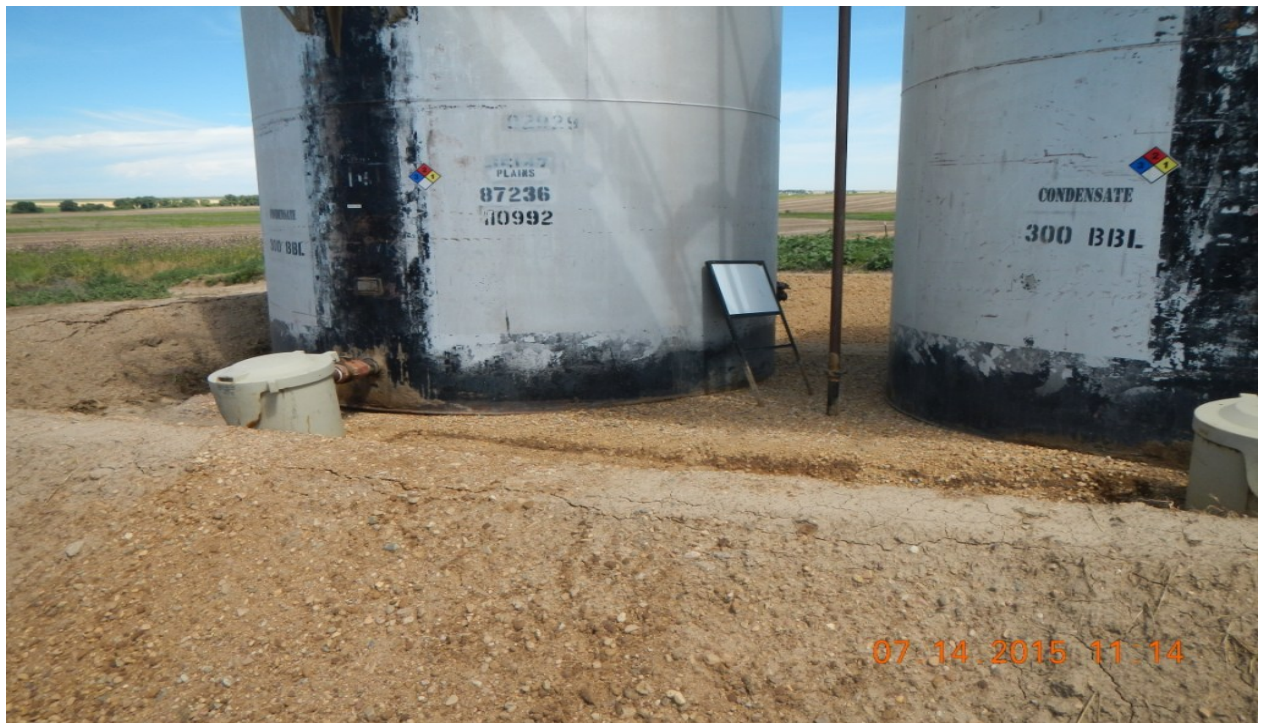
photo 2: Tank battery sign found leaning against the tank.
