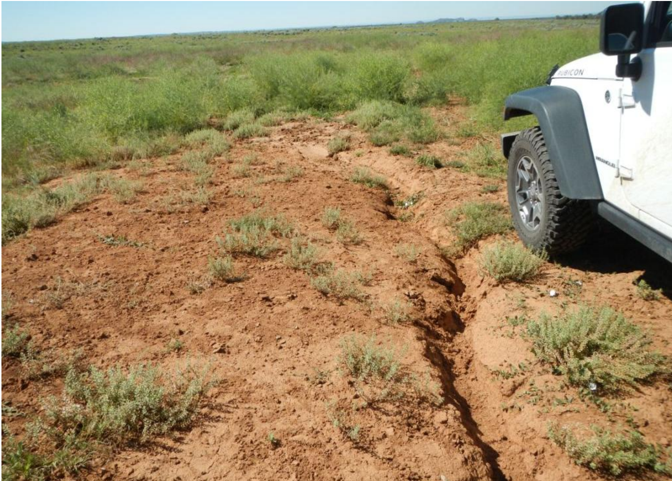
Photo 1. View of rill erosion (approximately 6 inches wide and 6 inches deep) at the entrance to the well pad.
