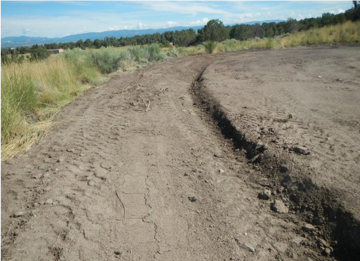
Photo 1. View of newly installed diversion along western edge of working area.
