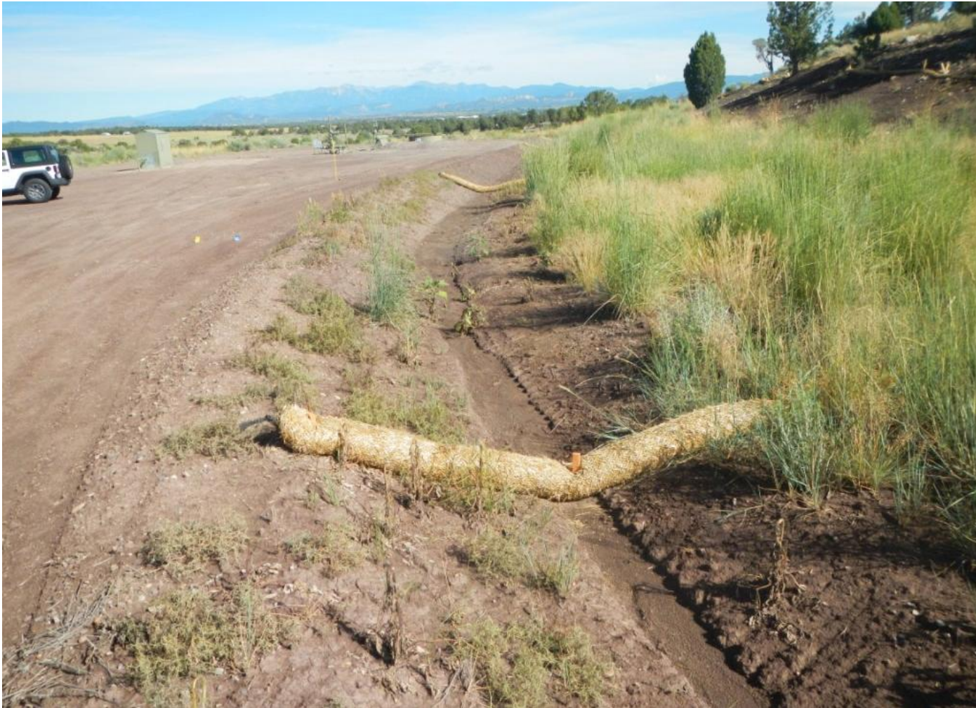
Photo 5. View of newly installed straw wattles within eastern diversion.
