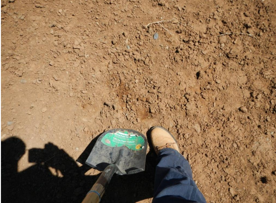
Photo 4. View of soil compaction within the project area (photo on left). Shovel cannot easily break soil. Can only dig approximately 2 to 3 inches.
