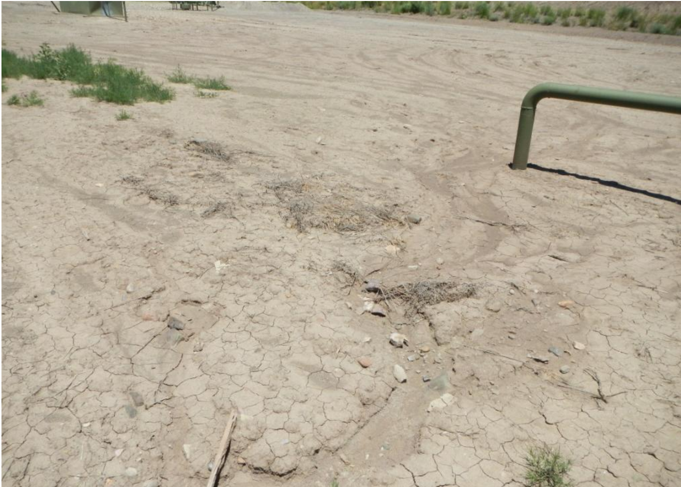
Photo 3. View of another erosional channel forming on well pad where concentrated stormwater flows off of the project area.
