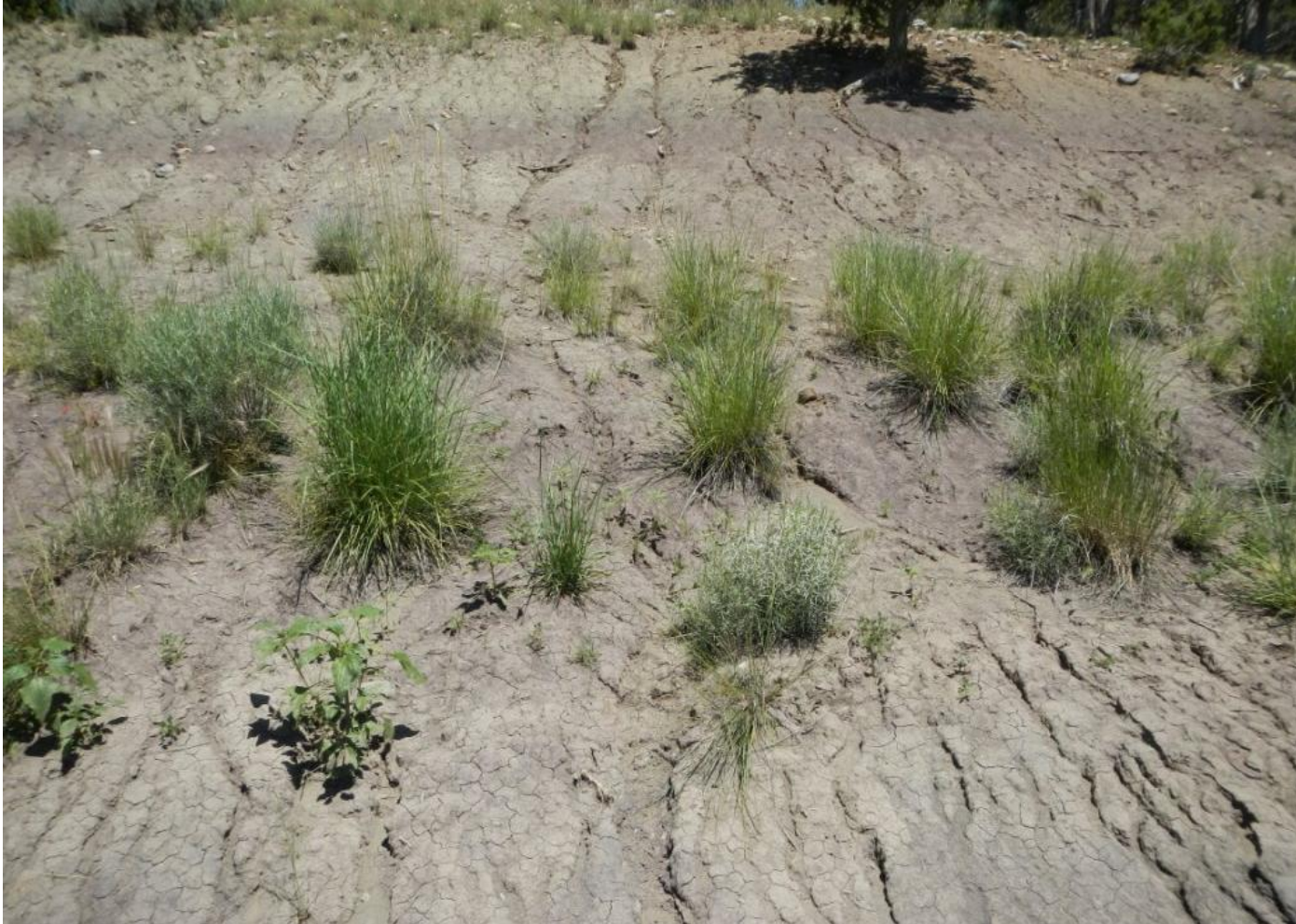
Photo 7. View of rill erosion within the eastern portion of the project area. Deep rills and significant sediment deposition at the toe of the slope are evidence that cut-slopes are not sufficiently stabilized.
