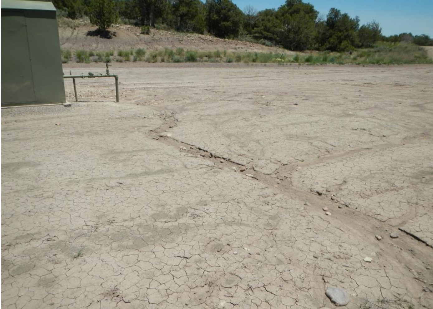
Photo 1. View of erosional channel forming within the well pad and flowing toward the southwestern portion of the project area.
