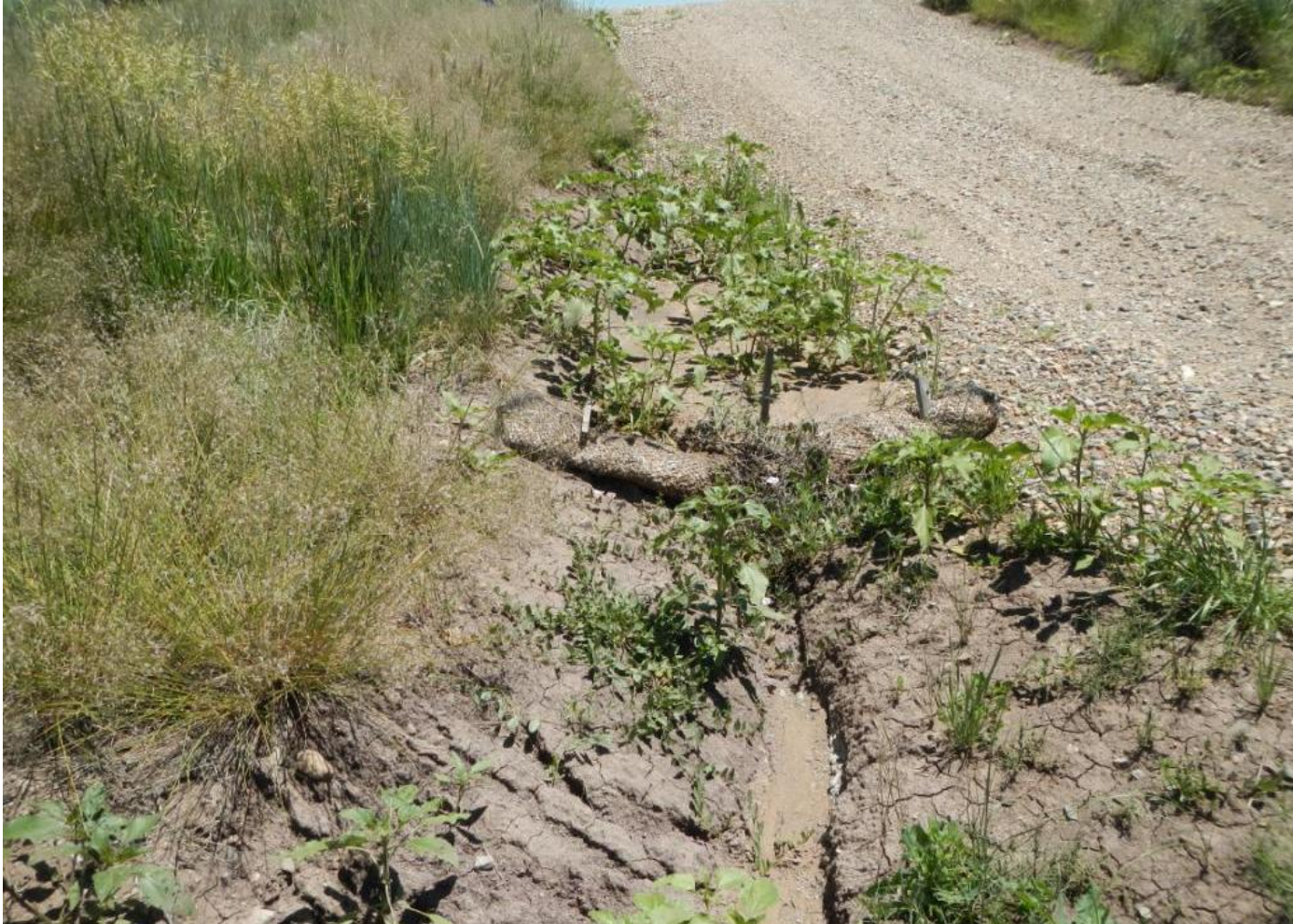
Photo 8. View of straw wattle along access road that is filled with sediment. It doesn't appear that this single straw wattle is a sufficient BMP to contain sediment flows along the access road.
