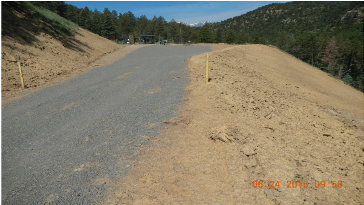
photo 3: Gravel has recently been spread on pad surface and location has recently been reclaimed.
