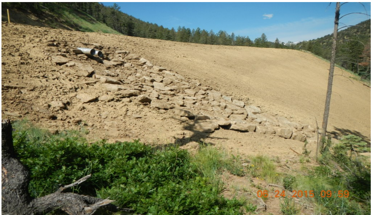
photo 4: Northeast corner of the location facing west. Culverts and rock outlet have been installed.
