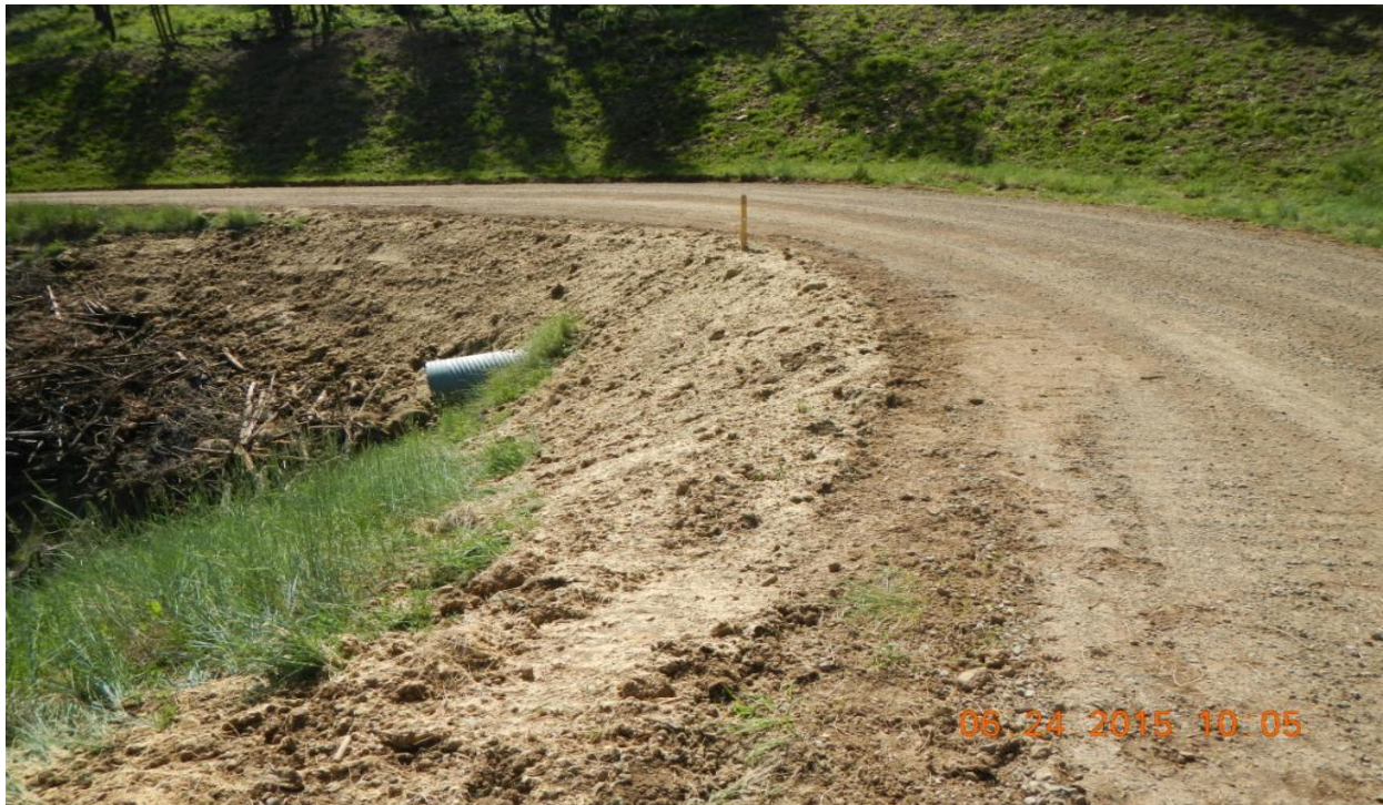
photo 9: Areas along the access road have recently been hydro mulched/seeded.
