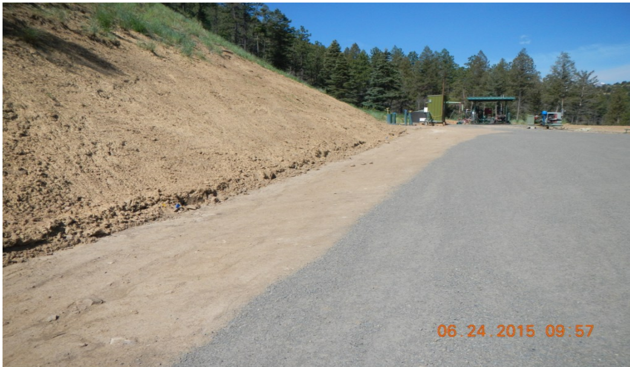
photo 8: Slope along the south side of the location has been hydro mulched/seeded.
