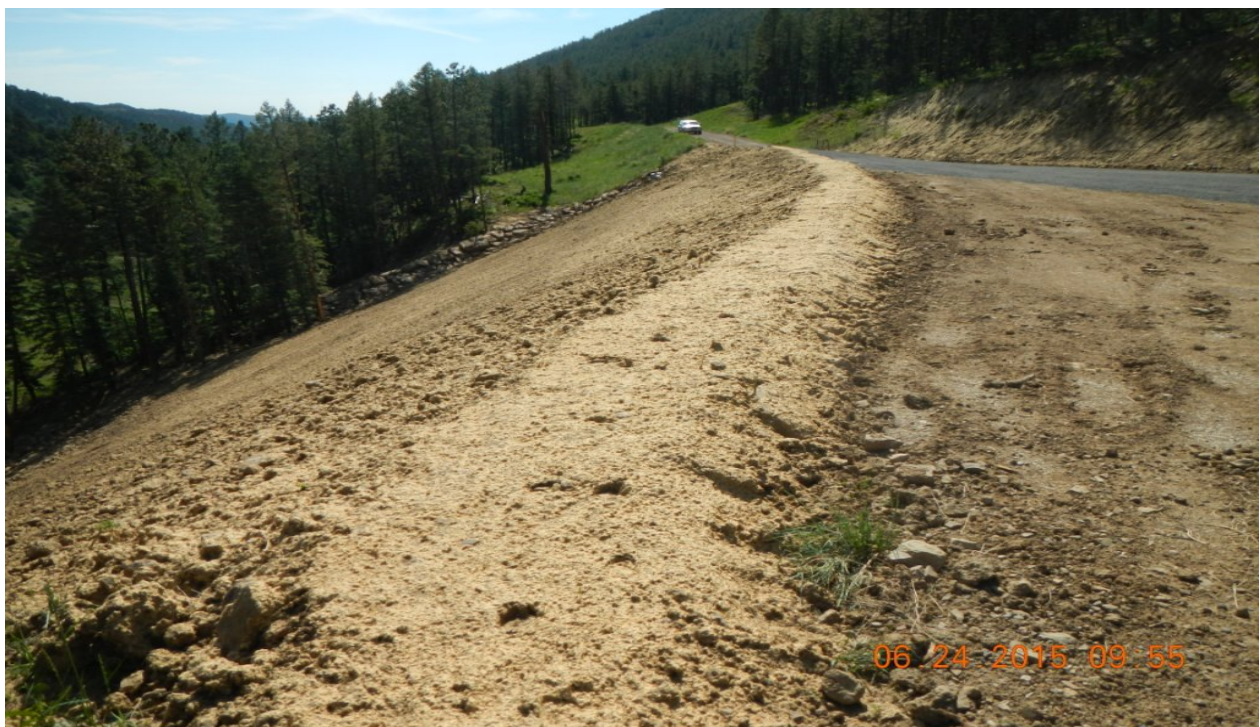
photo 6: Northwest corner of the location facing east. Slope has recently been hydro mulched/seeded.
