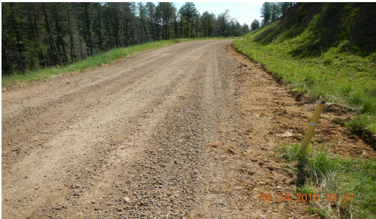
photo 10: The access road has recently been graded.
