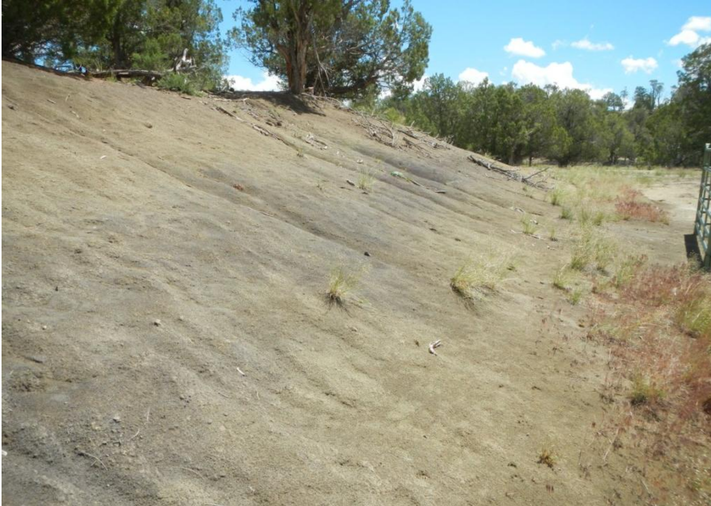
Photo 5. View of northern cut slope from northeastern edge facing eastward. Little vegetation on the slope. Indian ricegrass ( Achnatherum hymenoides ) and cheatgrass ( Bromus tectorum ) are growing in the eroded sediment at the toe of the slope.
