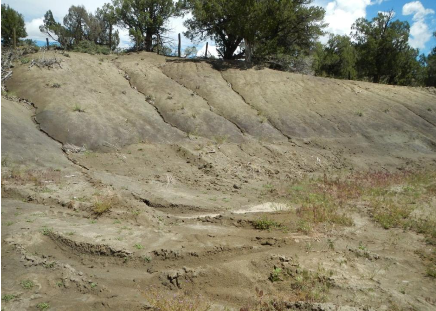
Photo 4. View of unprotected cut-slope in northwestern corner of project area. Rill erosion is apparent and little vegetation is established on the slope. Sediment that appears to have eroded off of the slope is visible in the foreground of the photo.
