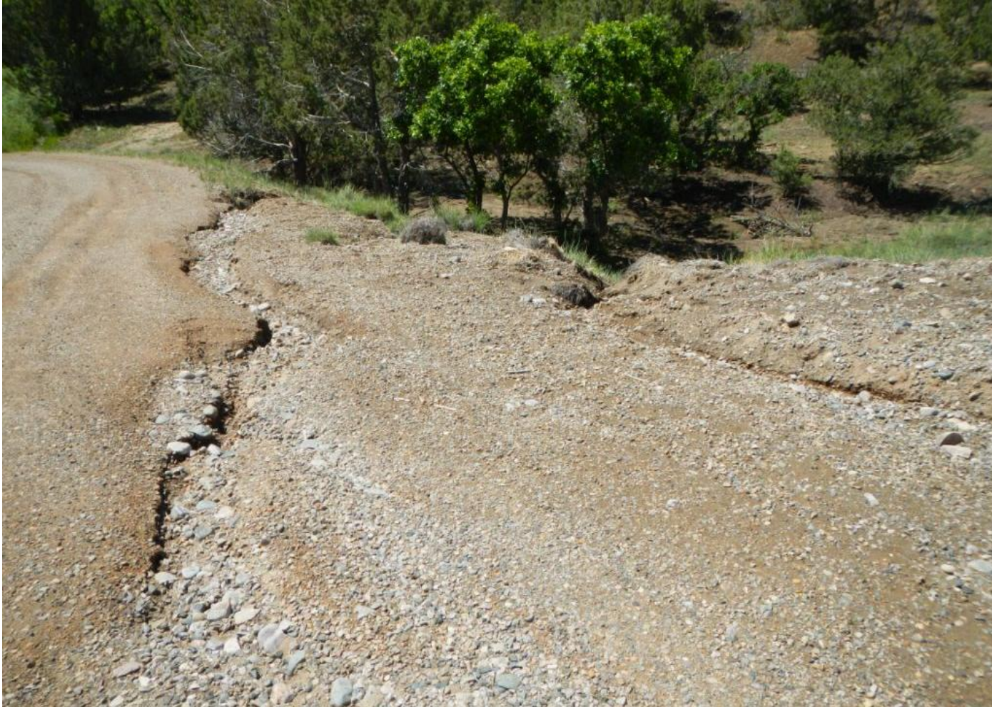
Photo 2. View of erosional channels approximately 1 to 2 feet wide and 1 to 2 feet deep in western edge of access road and southern portion of well pad.
