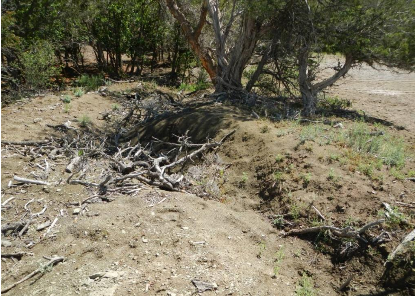
Photo 4. View of northern diversion channel facing downslope (eastward) toward the irrigation ditch. Stormwater BMPs are needed here to de-energize flows and filter sediment.
