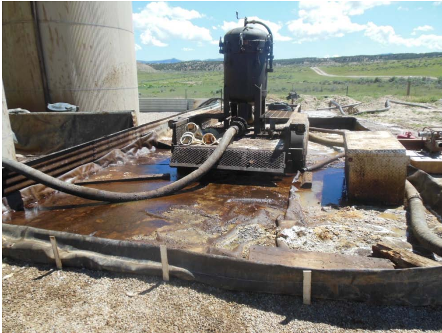
Secondary containment with excess fluid
