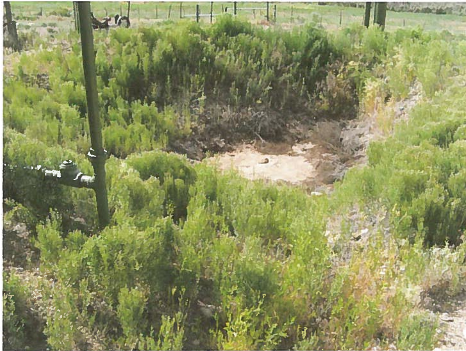
Star compressor condensate tank blowdown pit – June 22, 2007 Note weeds and general lack of maintenance
