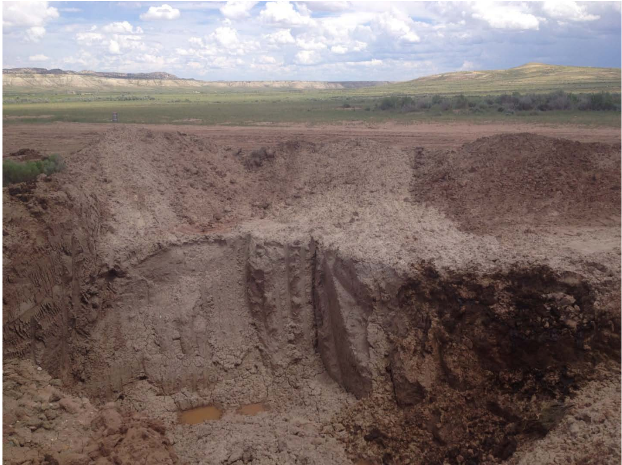
Area of pit id 100601, Approximate size 20' diameter, 15' deep. Approximate location is 40.979746, - 108.308608. Picture is looking north-west. Note; obvious hydrocarbon contamination.
