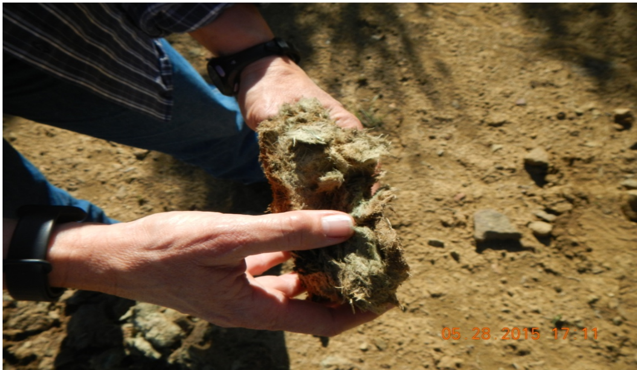
photo 8: Hydro mulch may have been applied to thick which may have impeded plant growth in this area.
