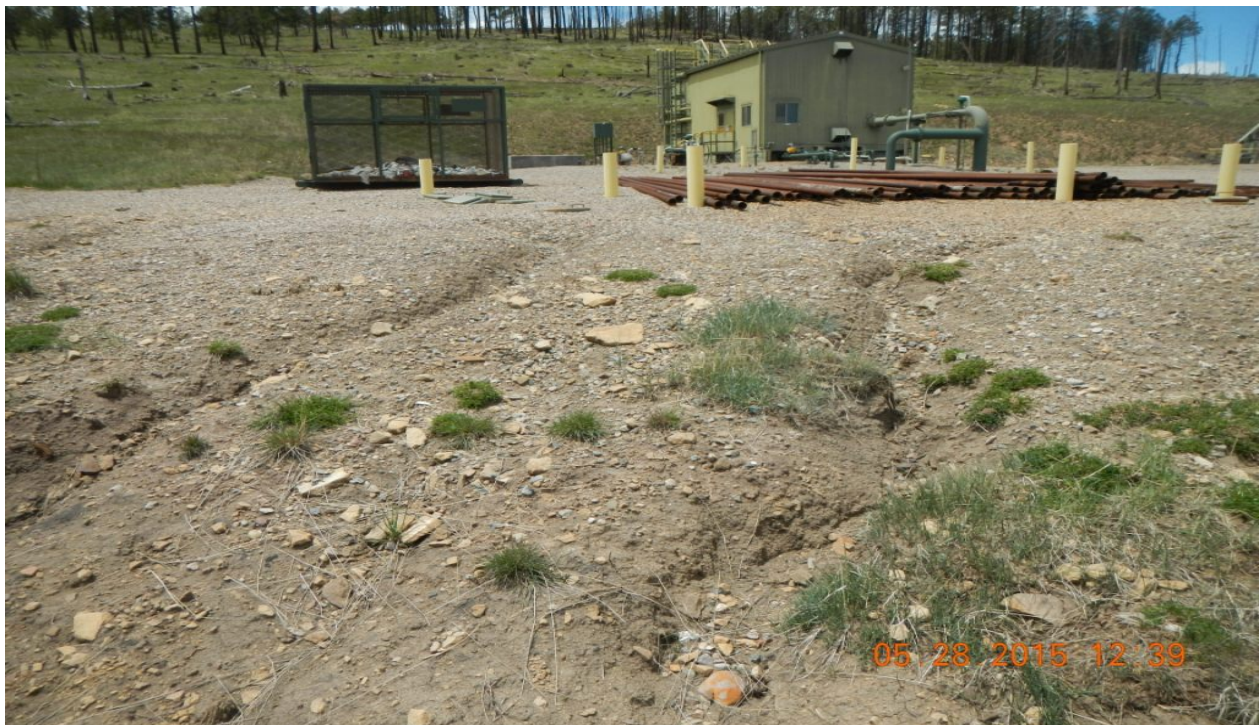
photo 2: Southeast side of location facing west. Erosion channels have formed along the east side of the pad.
