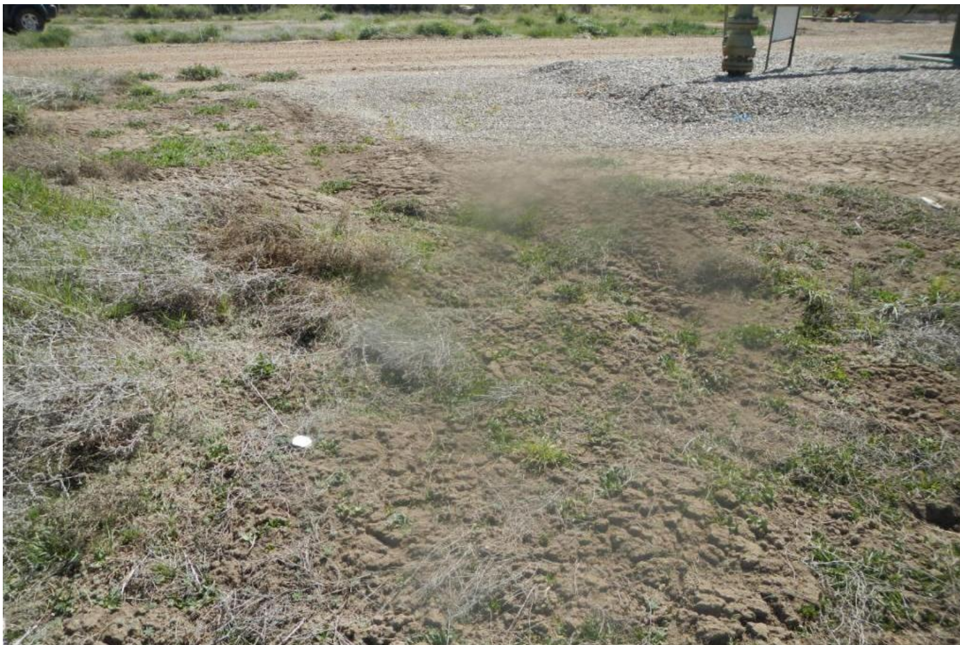
Photo 2. View of rill erosion from northern edge of the working area of the well pad.
