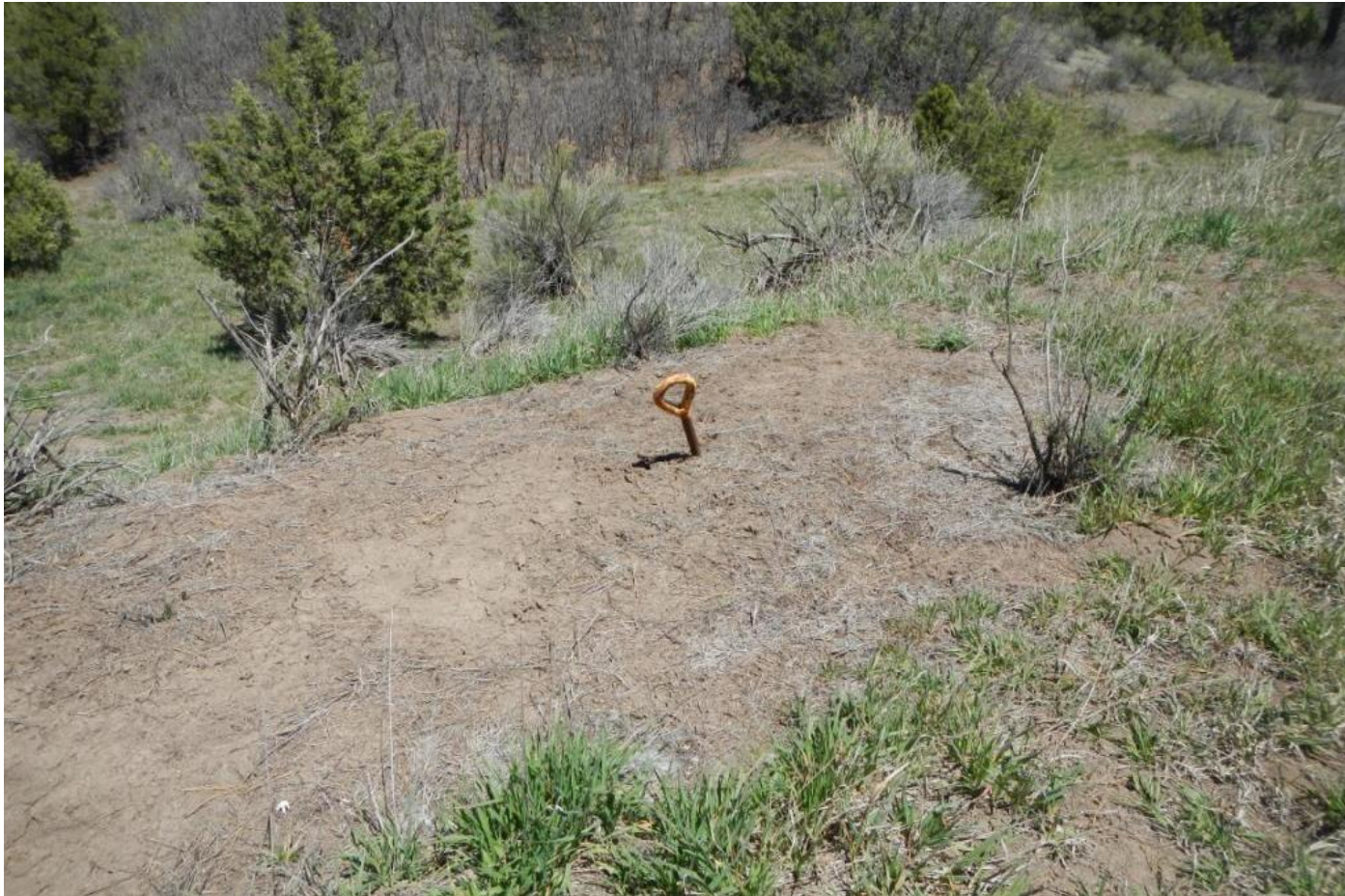
Photo 3. View of unmarked rig anchor.
