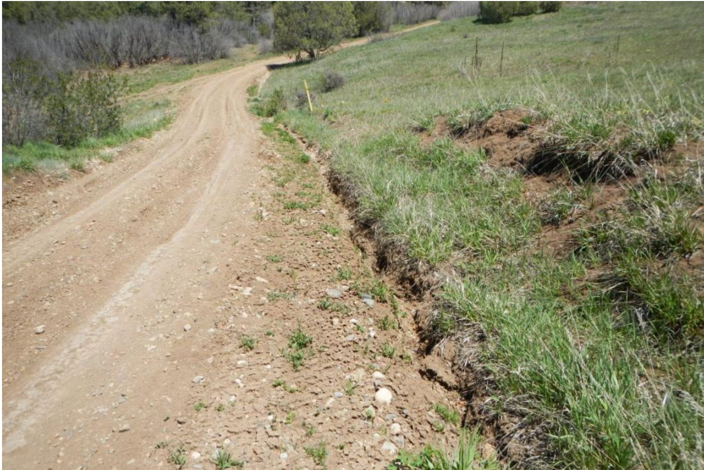
Photo 9. View of stormwater erosional channel forming along the edge of the access road.
