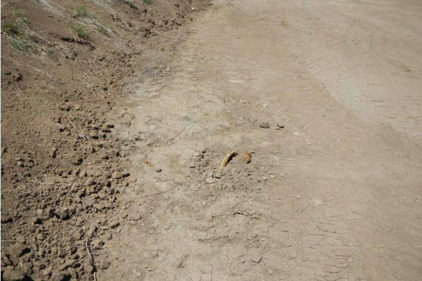
Photo 5. View of rig anchor that needs to be marked or removed.
