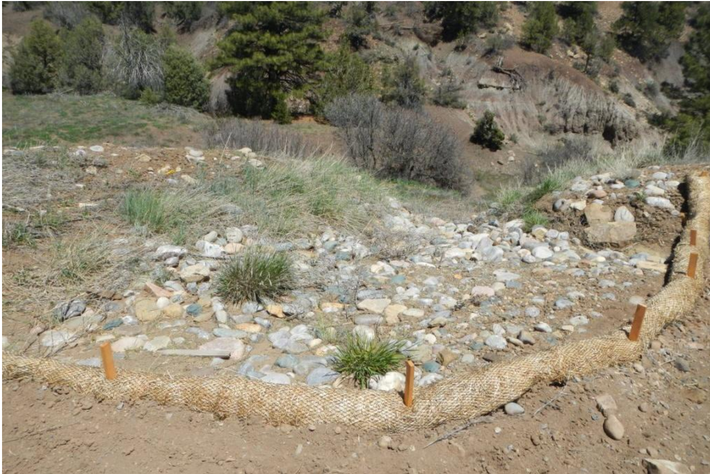
Photo 4. View of stormwater BMP within northern portion of interim reclamation area appears to be in good condition and functioning properly.
