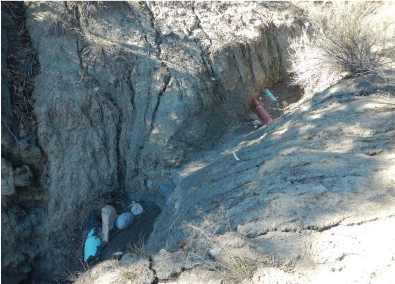
Photo 17. View of exposed pipeline below culvert outlet (approximately 2.5 miles on La Posta Road).
