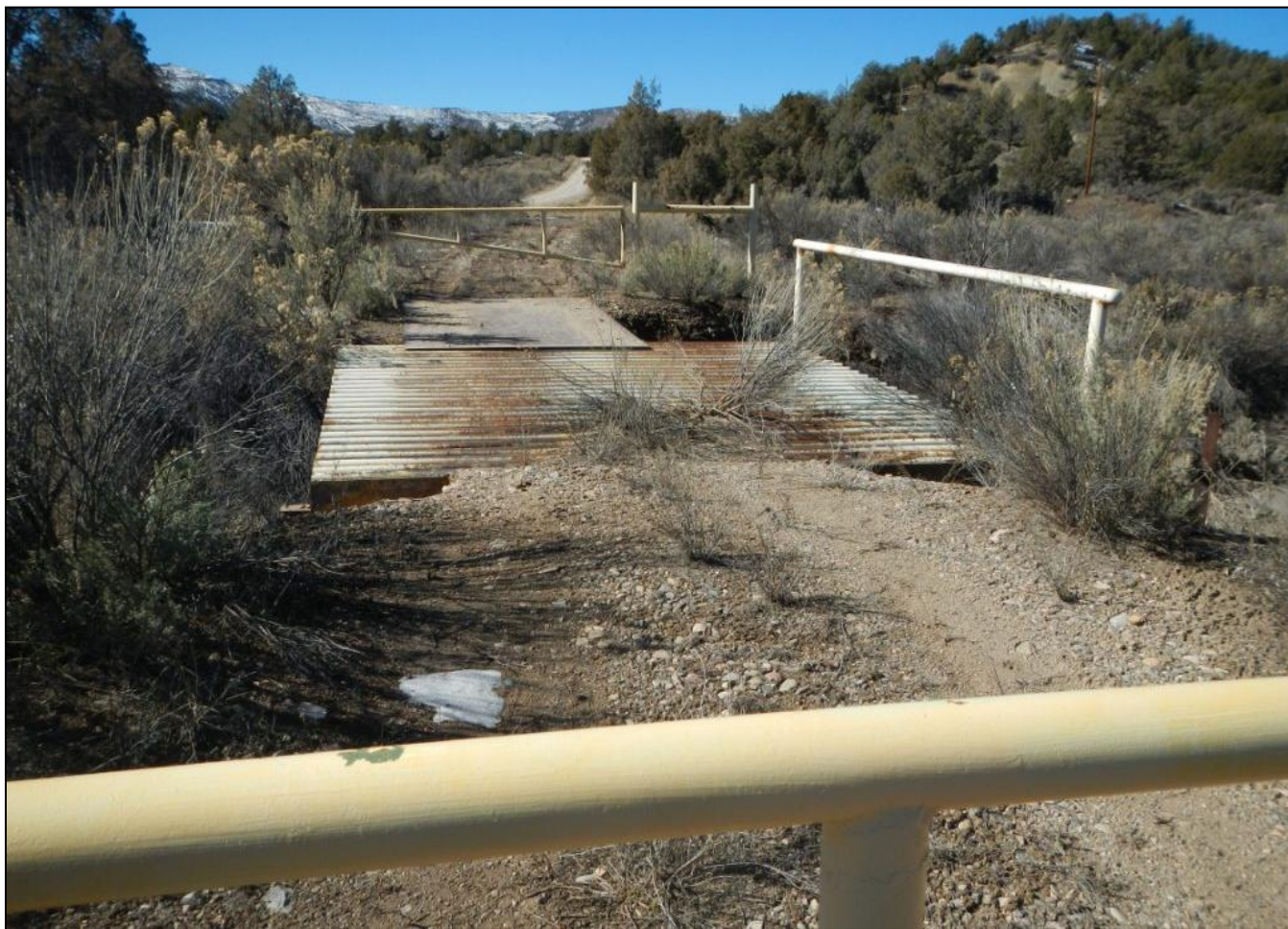
Photo 15. View of driving surface of old bridge at low water crossing.
