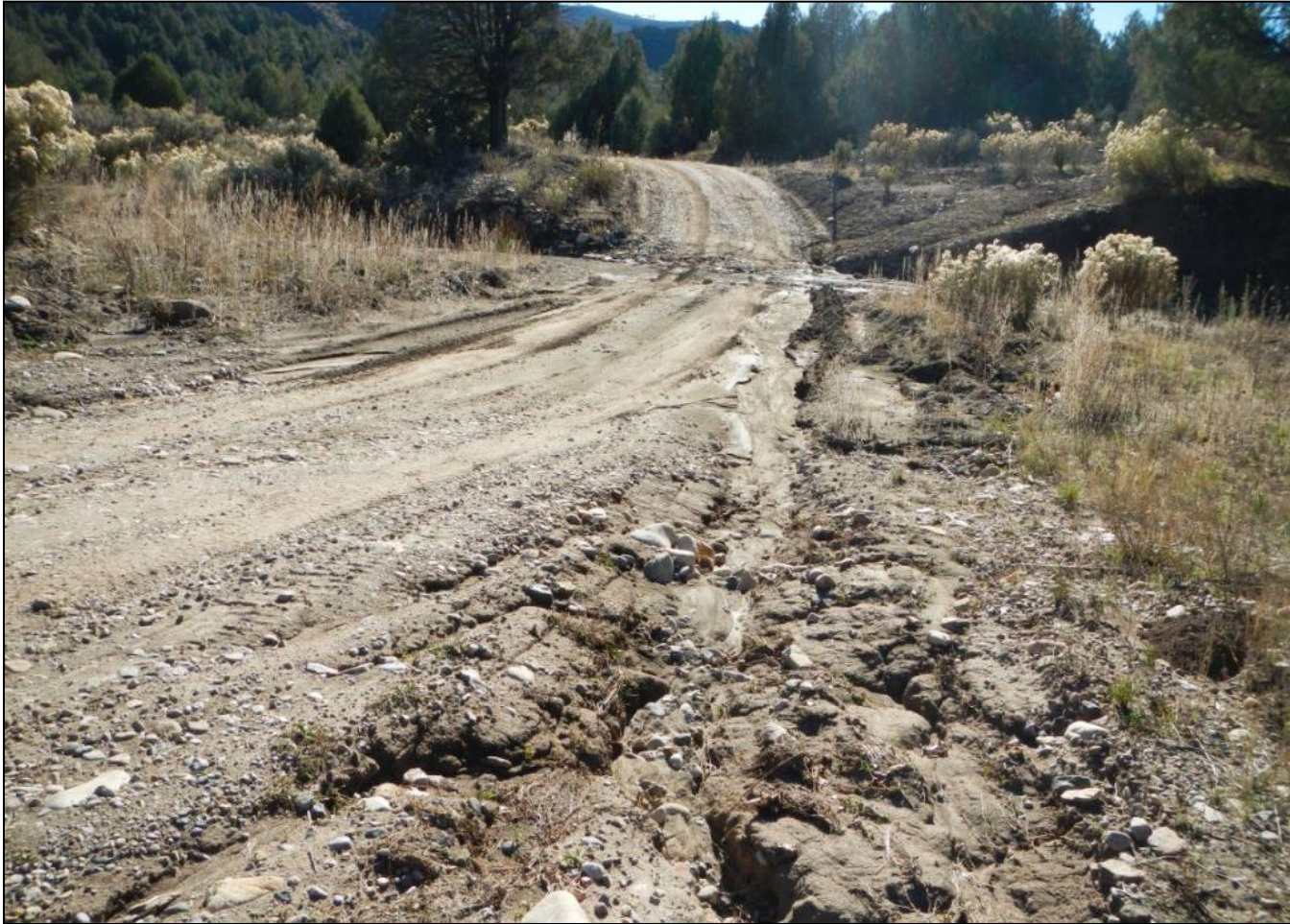
Photo 20. View of erosion on Hermit Haven Road flowing toward low water crossing. Turn off for Hermit Haven Road is approximately 3.4 miles on La Posta Road.
