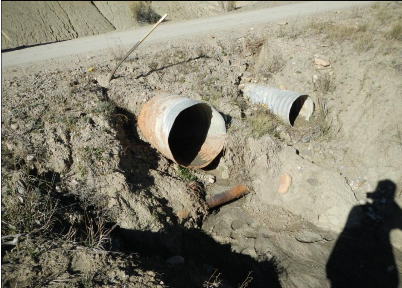
Photo 16. View of exposed pipeline at culvert outlet (approximately 2.5 miles on La Posta Road).
