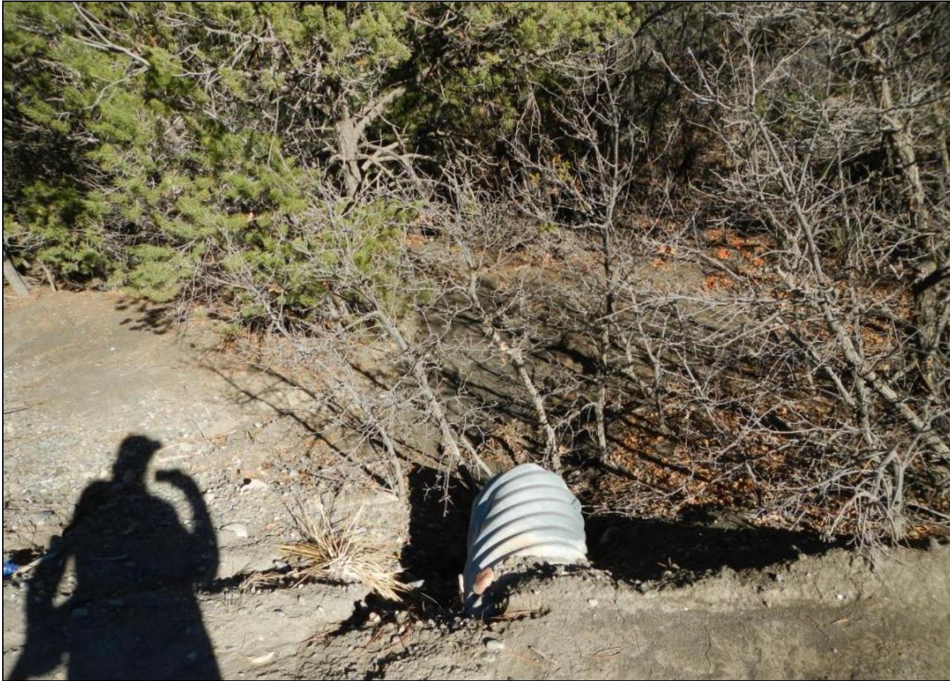
Photo 18. View of culvert outlet directing flows onto private property outside of normal flow pattern at approximately 3.0 miles on La Posta Road.
