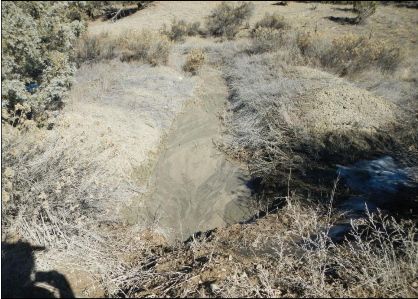
Photo 10. Culvert outlet at 1.4 mile on La Posta Road. Outlet nearly 100 percent blocked by sediment.
