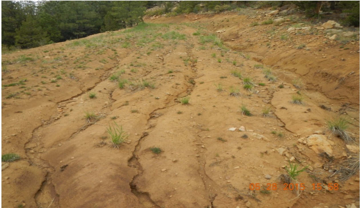
photo 3: No BMP's have been installed along the access road to prevent erosion from worsening.
