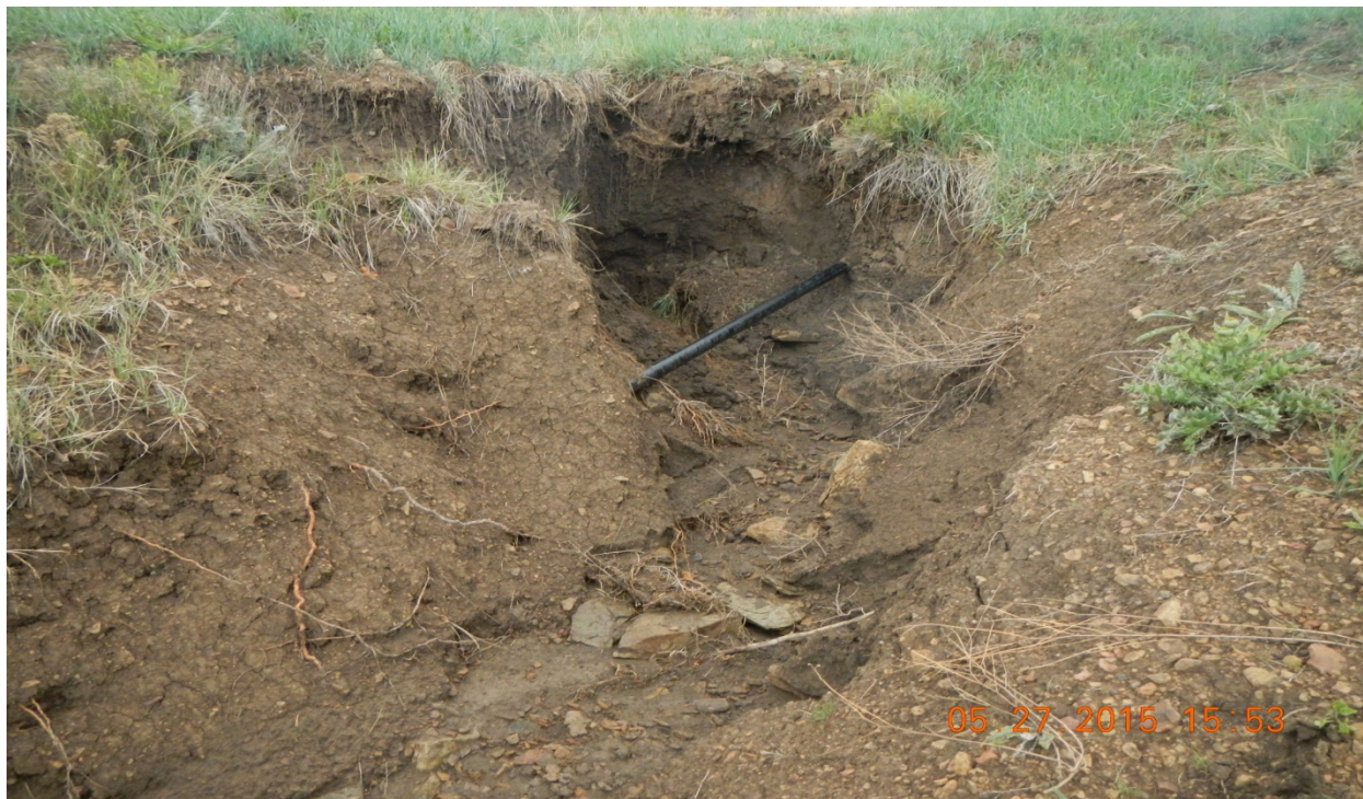
photo 11: Plastic pipe is exposed as a result of erosion which has occurred.
