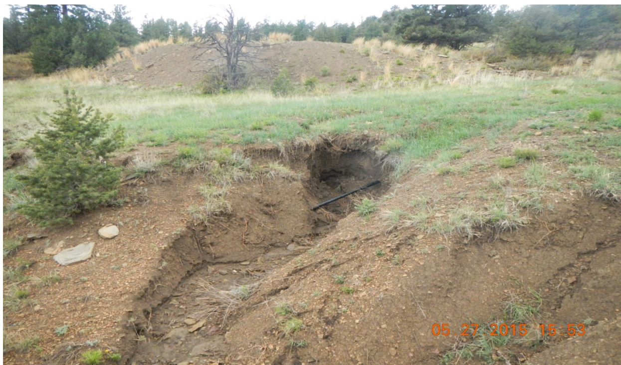
photo 10: Erosion occurring northeast of the pit area where water enters from the access road diversion ditch and pit disturbance area.
