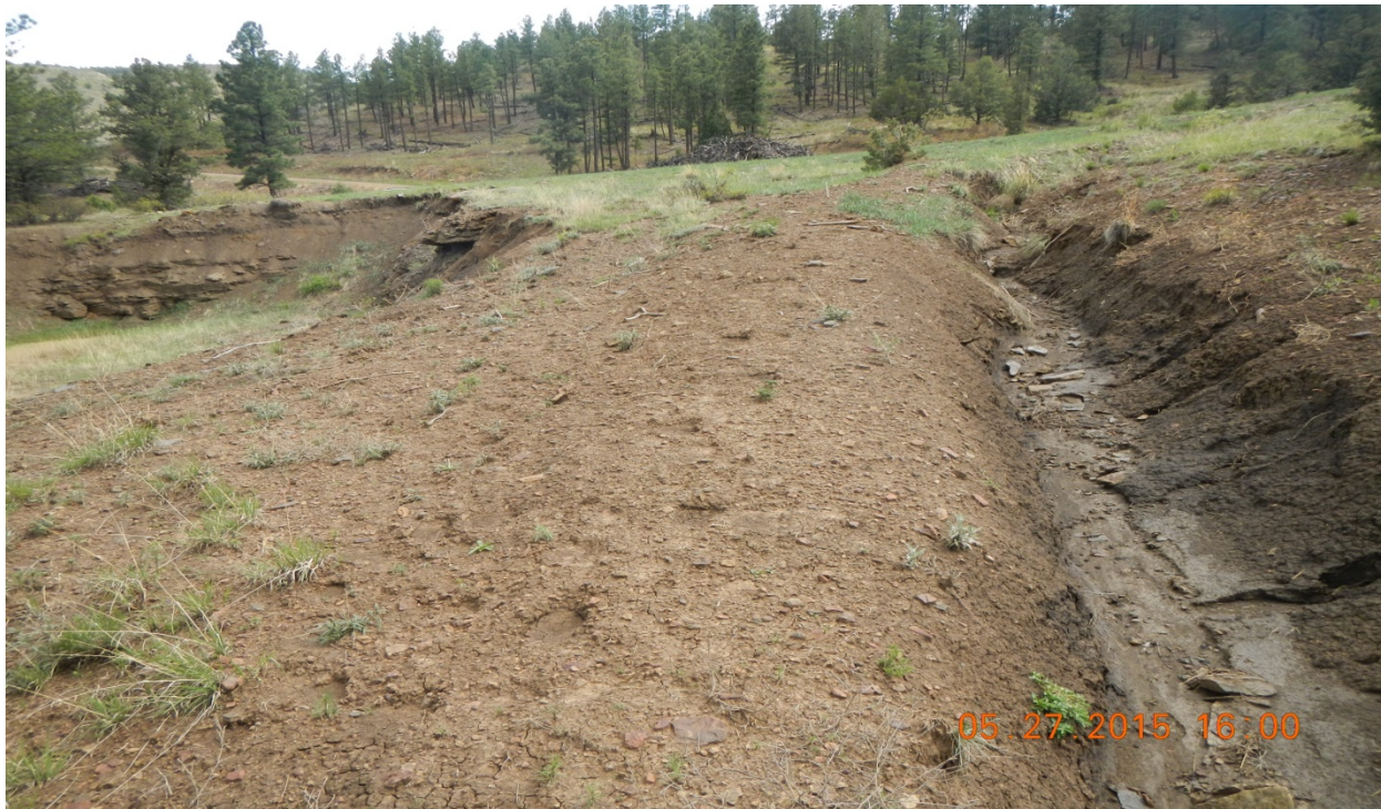
photo 5: Facing south. A diversion ditch from the access road diverts water around the west side of pit.
