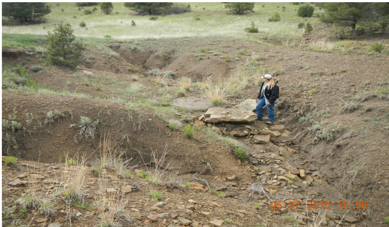
photo 12: Erosion gullies where water enters from the access road diversion ditch and pit disturbance area.
