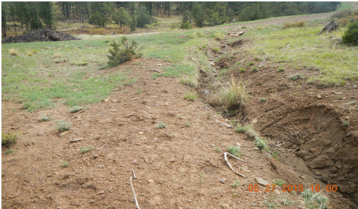
photo 6: The diversion ditch from the access road is being incised and needs BMP's installed to prevent erosion.
