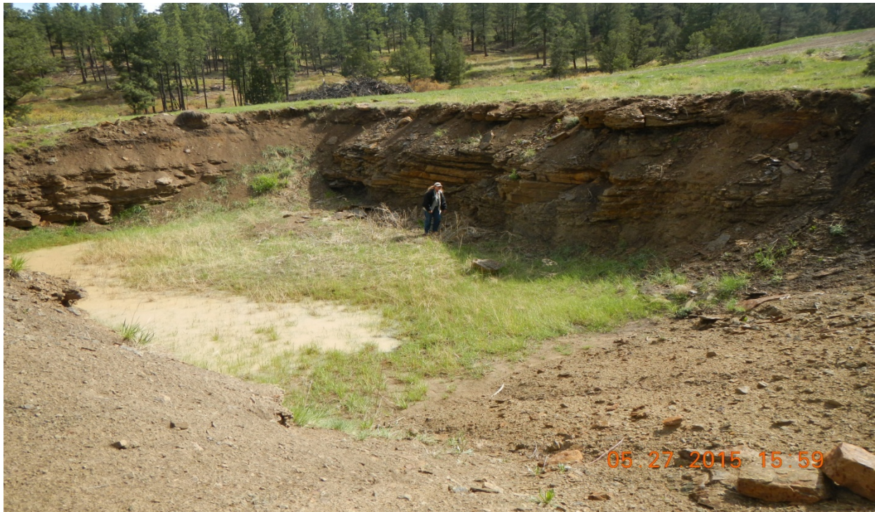
photo 3: Facing south towards the offsite pit. Three of the sides have unstable vertical cuts.
