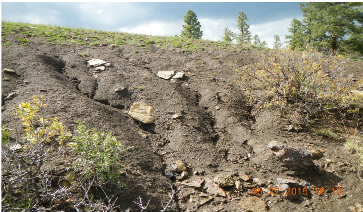
photo 6: The base of the pad where erosion is occurring.
