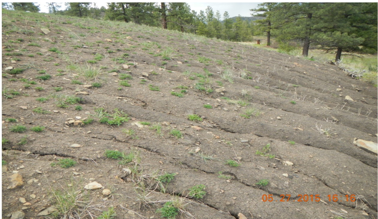
photo 4: Facing north along the east side of the location. Erosion channels have developed off the pad.
