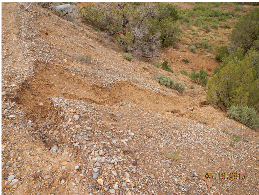
Erosion on side of access road.
