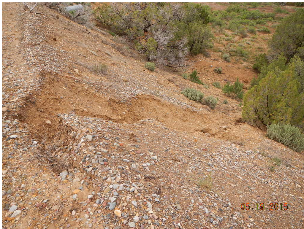
Erosion on side of access road.
