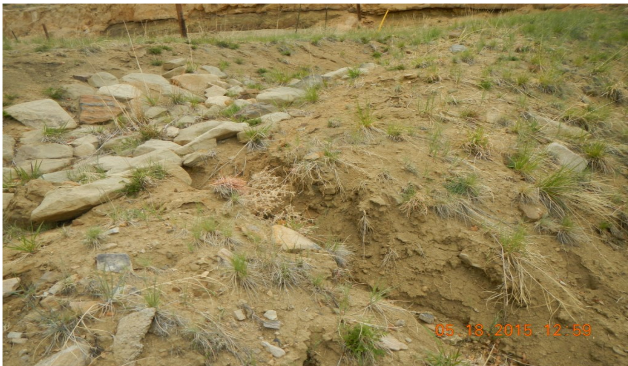
photo 6: Erosion channel has formed transporting sediment off the pad. See photo #5 for reference.
