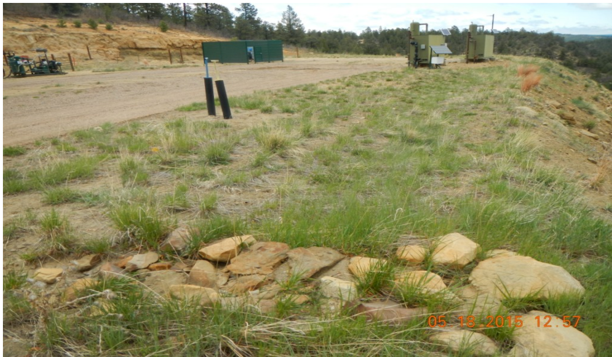
photo 3: Facing northeast towards the location
