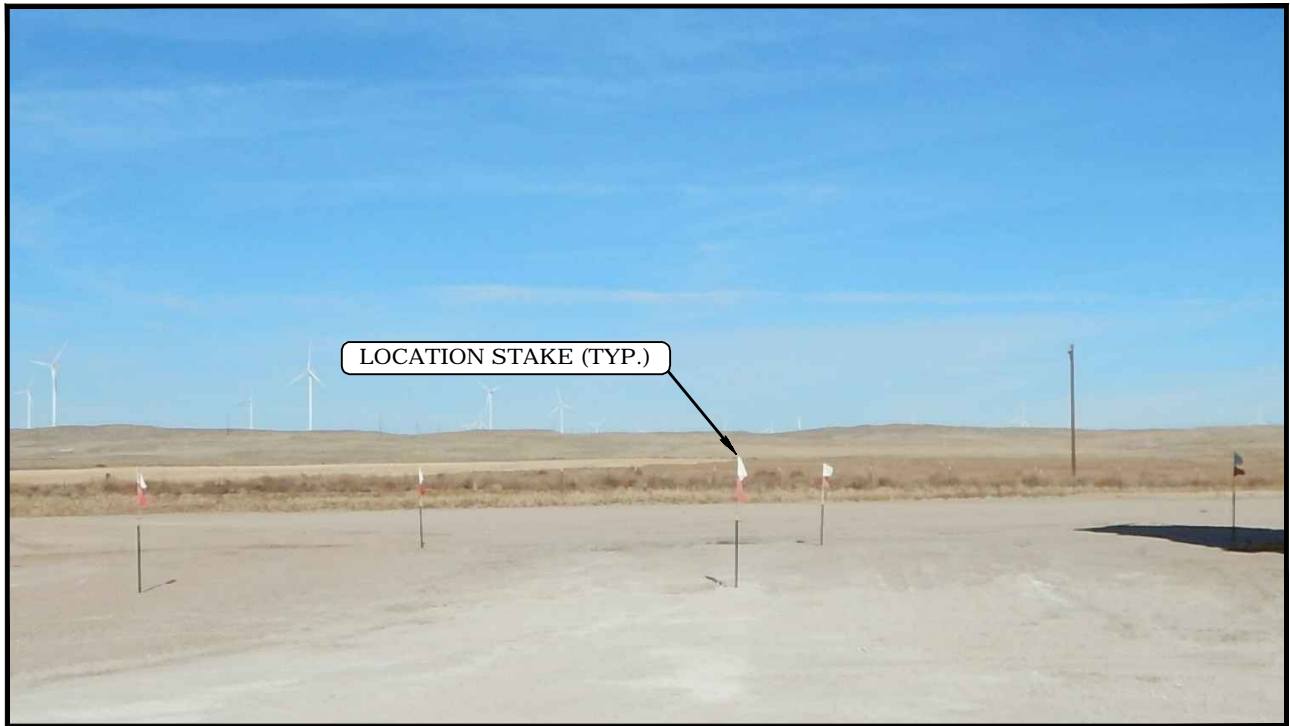
PHOTO: VIEW OF LOCATION STAKES
